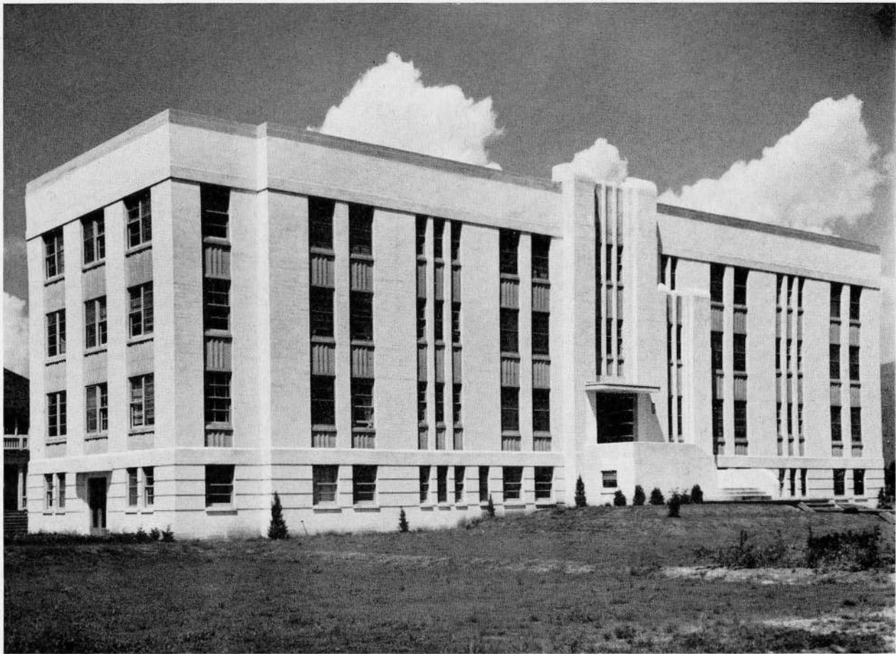
NEW CHILLIWACK GENERAL HOSPITAL, CHILLIWACK, BRITISH COLUMBIA
