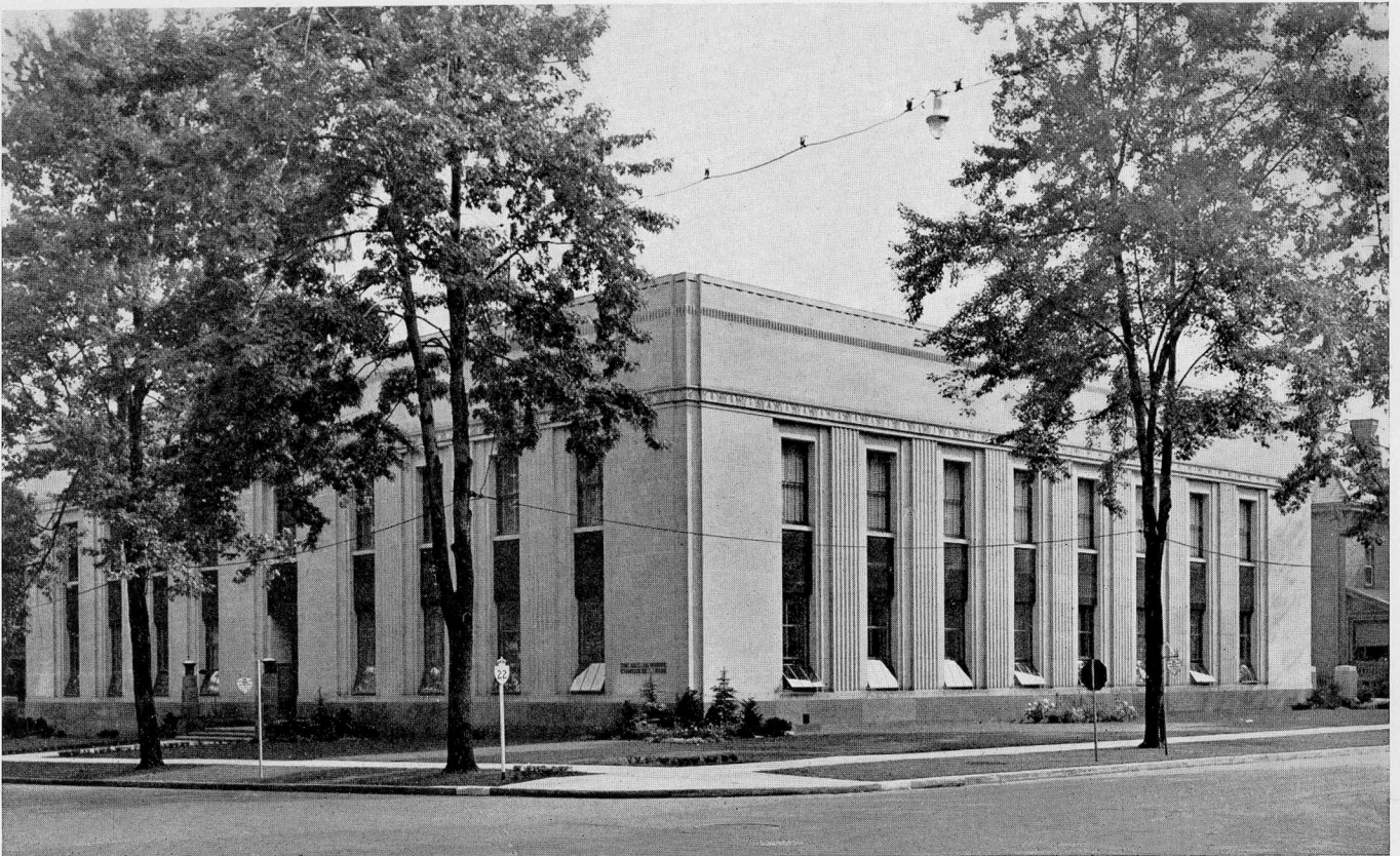
THE BELL TELEPHONE COMPANY OF CANADA, LONDON, ONTARIO
