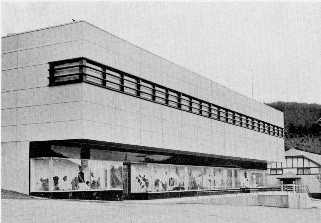
WALNUT STREET FACADE, showing the cantilever second floor, with louvered lights to second floor display. These windows, on second floor, were kept high so as to allow merchandise to be placed against this outside wall at a height of 6'6".
