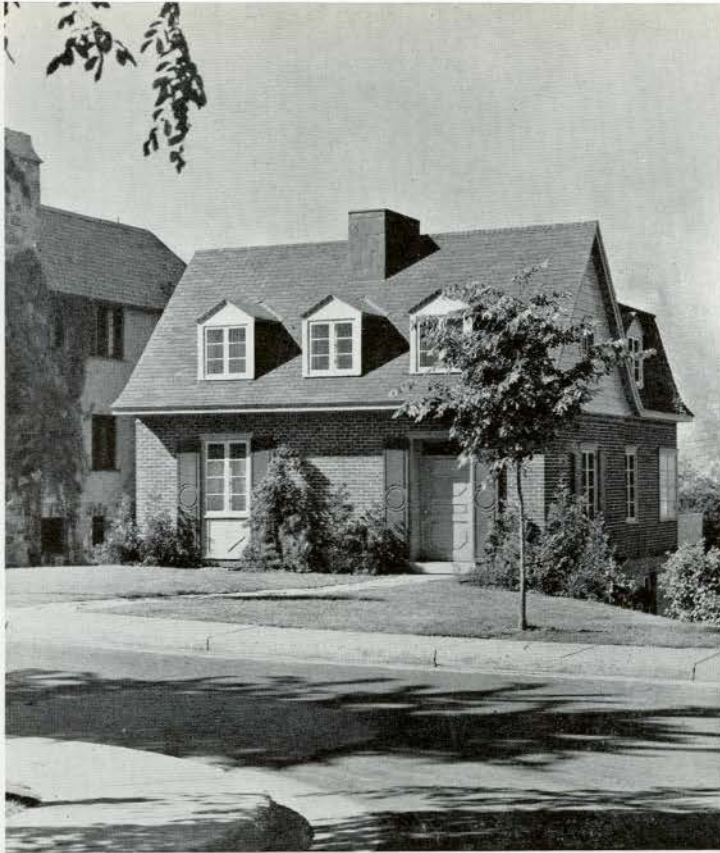
HOUSE OF MR. A. LESLIE PERRY, MONTREAL, QUEBEC PERRY, LUKE AND LITTLE, ARCHITECTS
