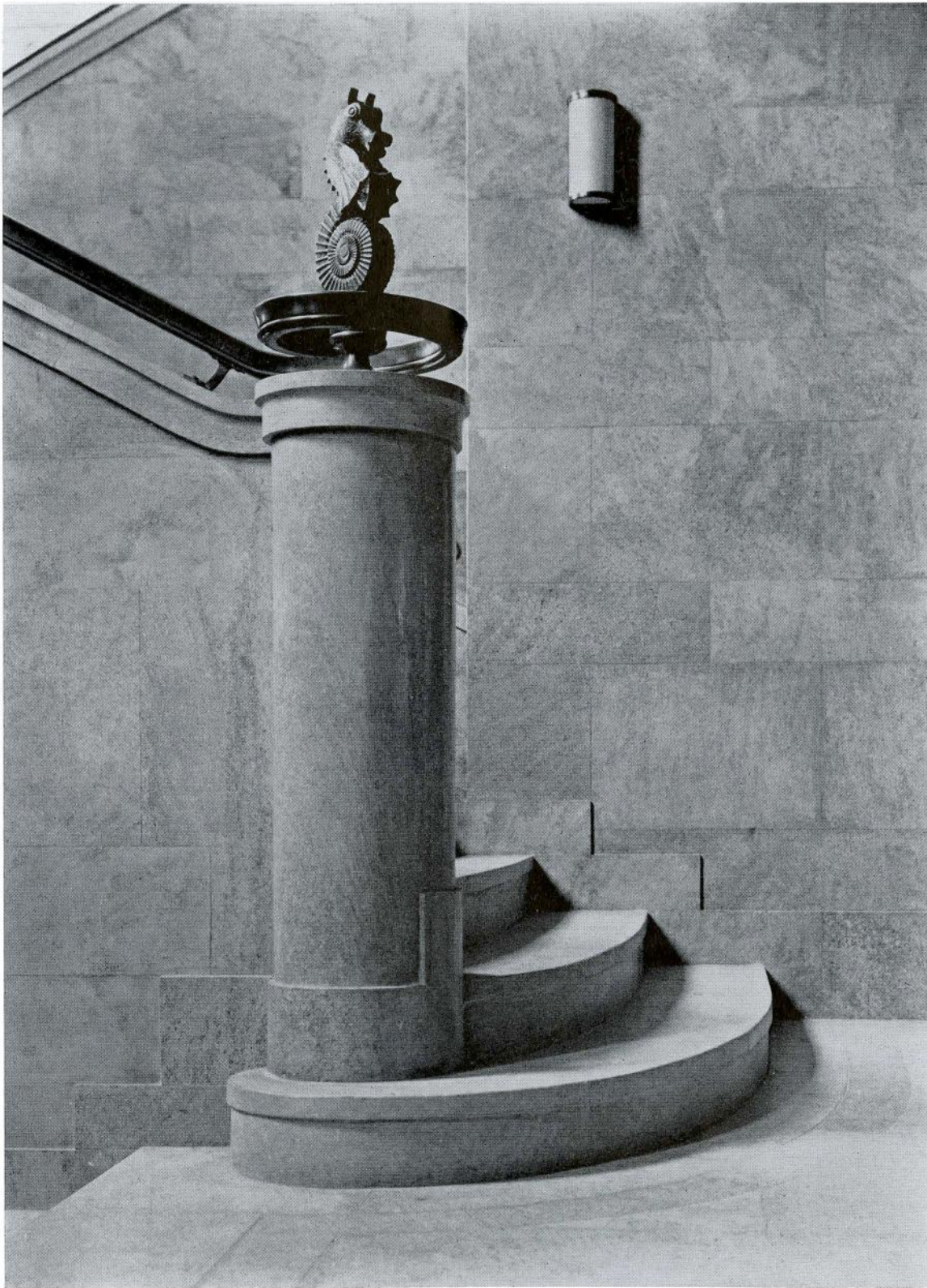
DETAIL OF NEWEL OF MAIN STAIRCASE
