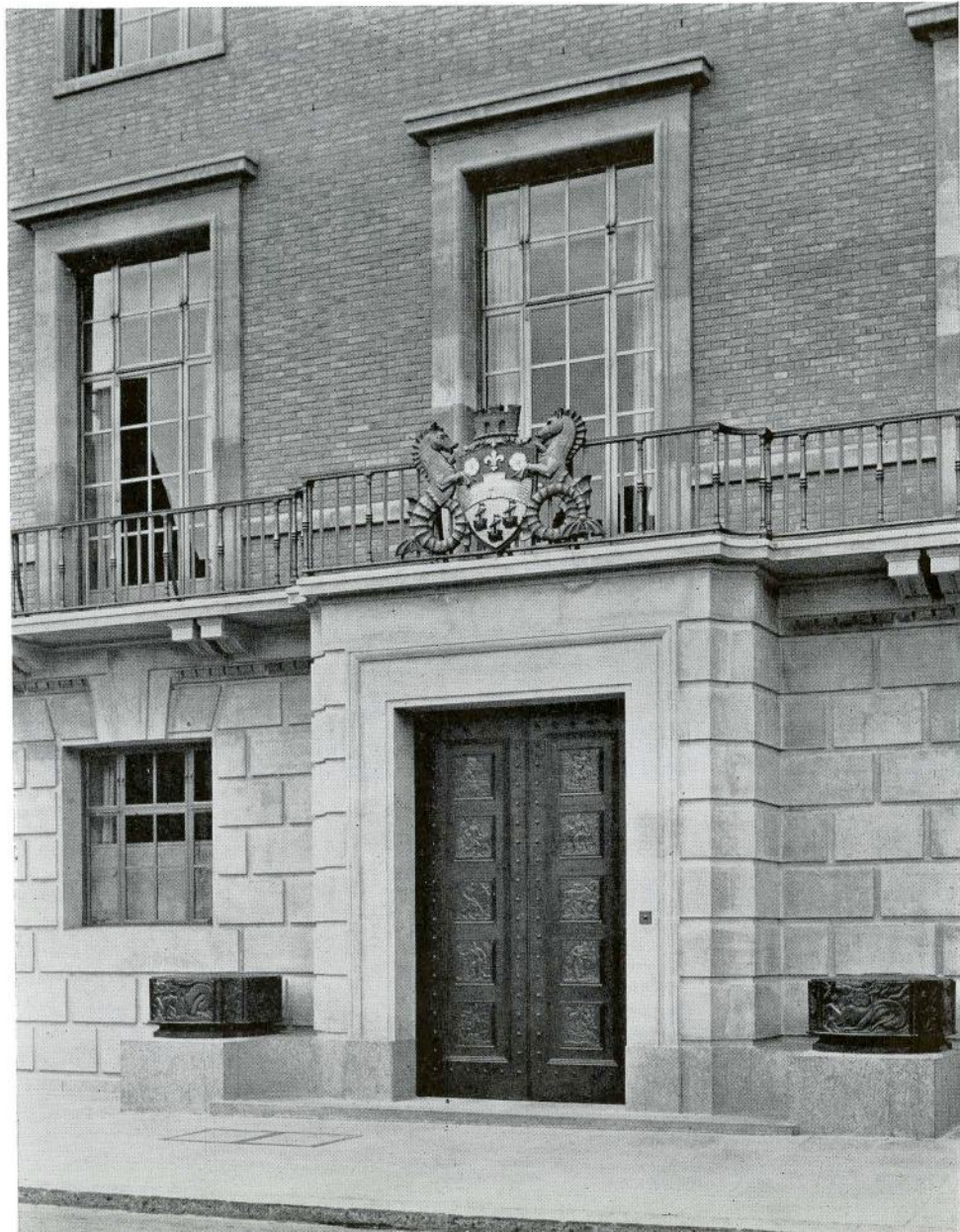
DETAIL OF MAIN ENTRANCE
