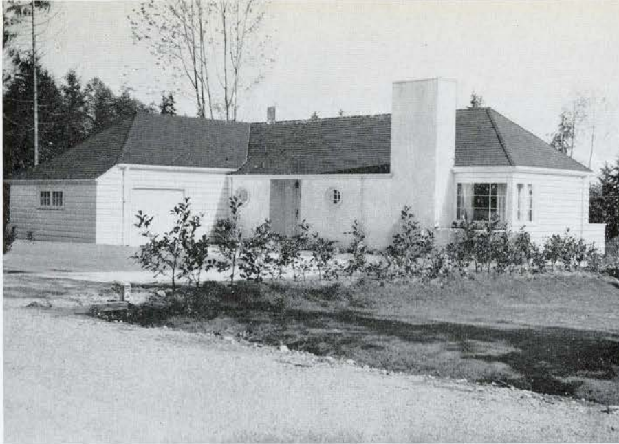
HOUSE OF MR. K. BLACK, WEST VANCOUVER, BRITISH COLUMBIA C. B. K. VAN NORMAN, ARCHITECT
