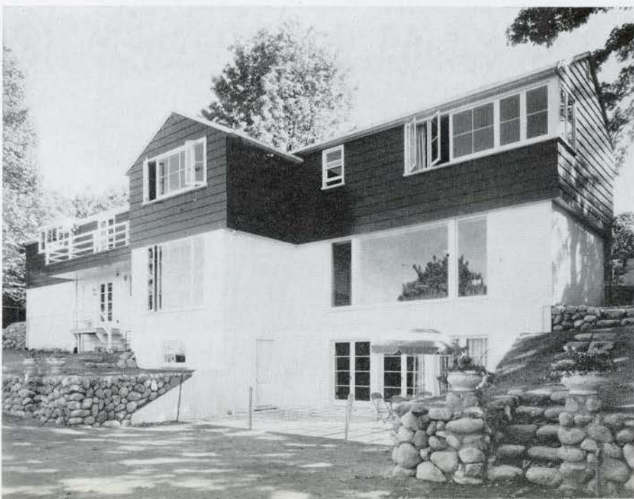
HOUSE OF MR. H. HACKING, VANCOUVER, BRITISH COLUMBIA C. B. K. VAN NORMAN, ARCHITECT
