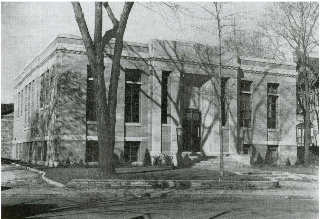
REGISTRY OFFICE FOR COUNTY OF WATERLOO, KITCHENER, ONTARIO RAY M. HALL, ARCHITECT
