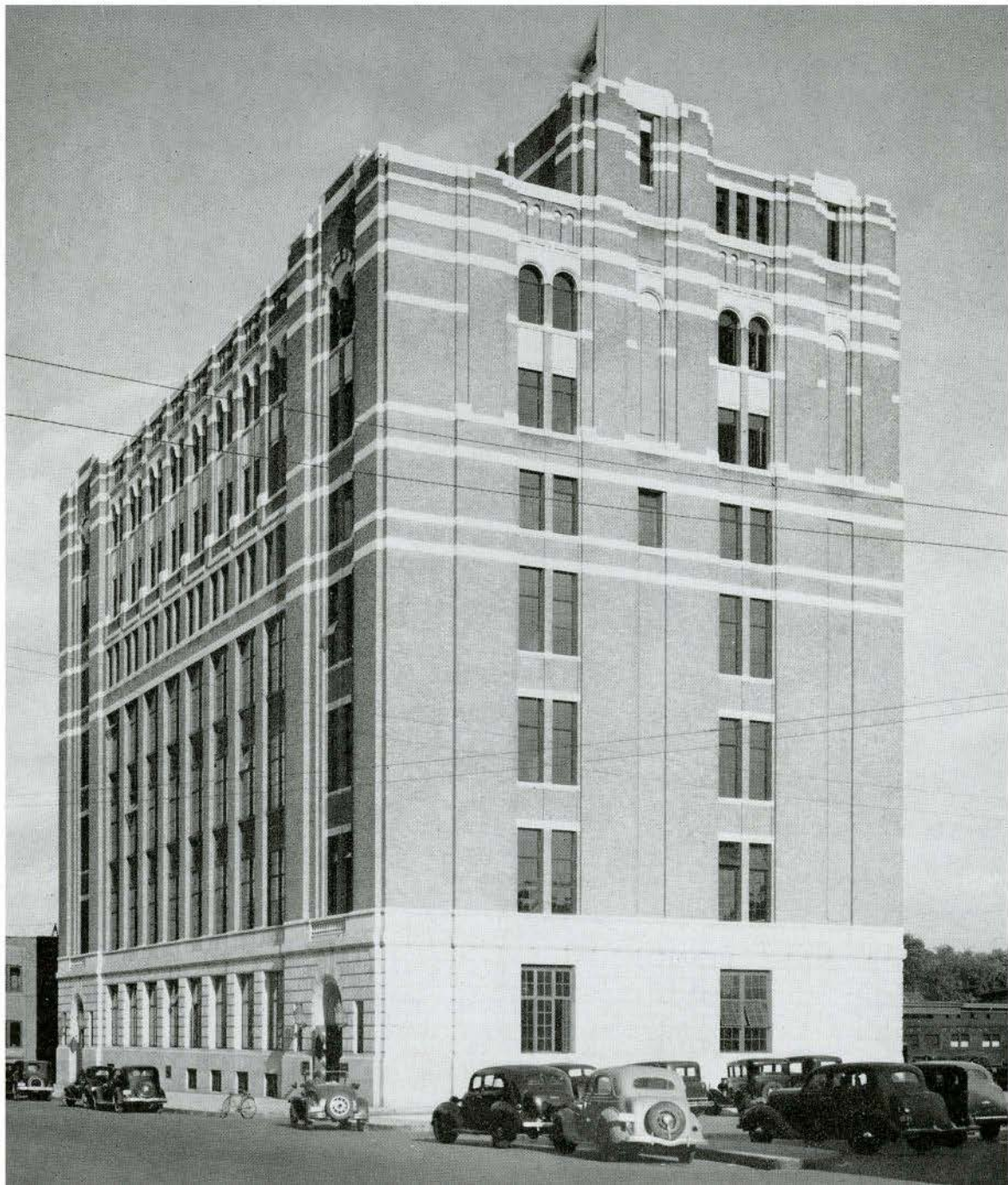
POSTAL TERMINAL BUILDING, OTTAWA, ONTARIO BURGESS AND GARDNER, ARCHITECTS
