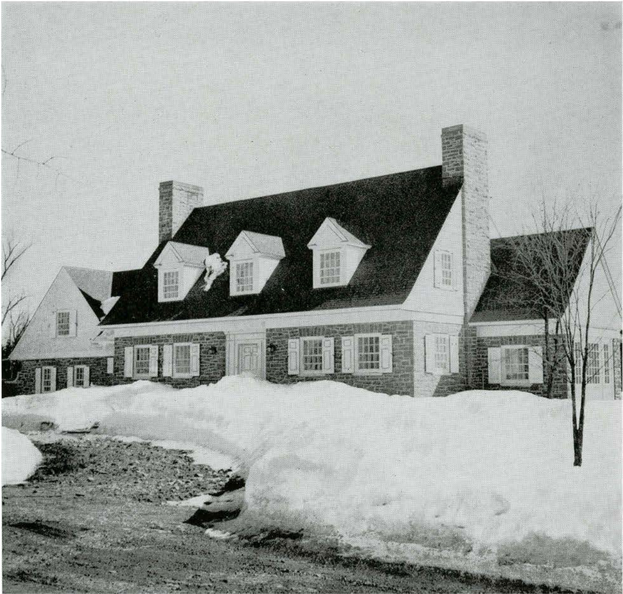
HOUSE OF MR. D. K. MacTAVISH, ROCKLIFFE PARK, ONTARIO ROPER, MORIN AND BELCOURT, ARCHITECTS
