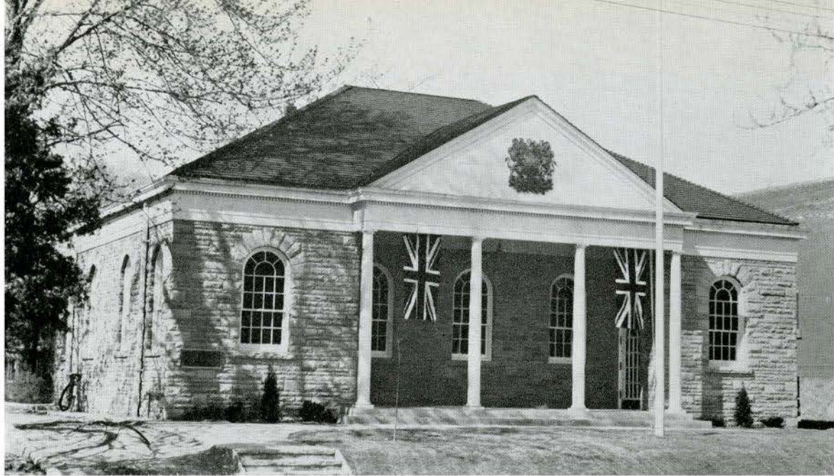
POST OFFICE, BURLINGTON, ONTARIO H. E. MURTON, ARCHITECT
