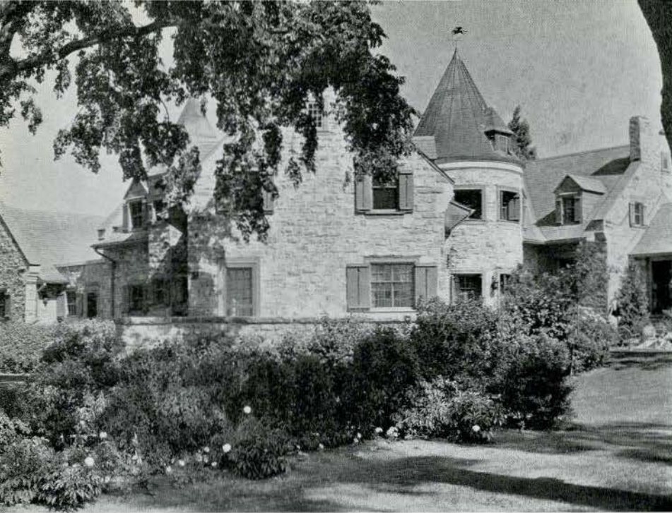
HOUSE OF MR. J. BOWMAN PECK, CAP ST. JACQUES, QUEBEC H. A. PECK, ARCHITECT
