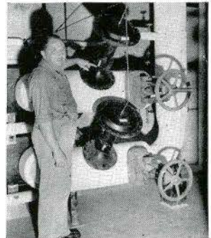
Upper left: Walt Disney (right) and Chief Engineer William E. Garity inspect the Johnson central control panel in the Camera Building. Above: Johnson valves on hot water heating mains in the Central Heating Plant.
