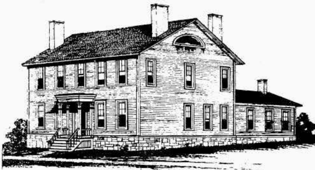
VIEW BEFORE ALTERATION
