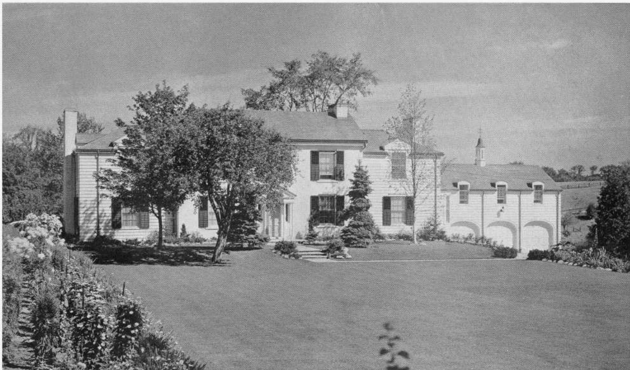
RESIDENCE OF H. L. NATHANSON, ESQ., TORONTO Wilkes and Fisher, M.M.R.A.I.C., Architects Award for Merit—Sixth Annual Exhibition of the Royal Architectural Institute of Canada
