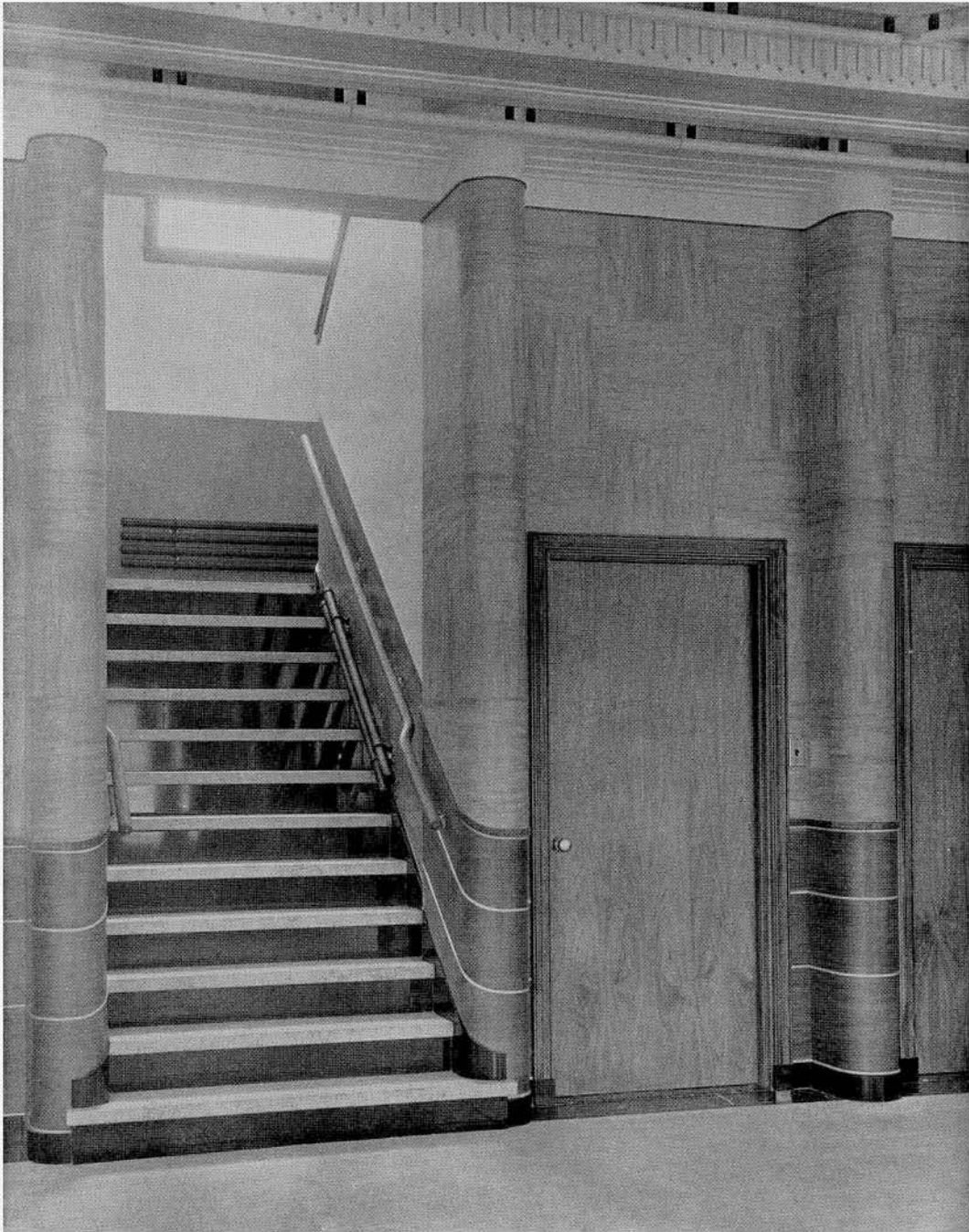
DETAIL AT REAR OF SHOWROOM—BUILDING FOR THE SHAWINIGAN WATER AND POWER COMPANY, SHAWINIGAN FALLS, P.Q.
