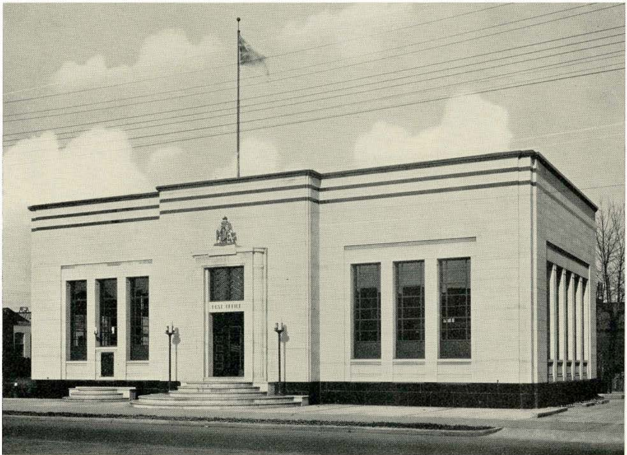
DOMINION PUBLIC BUILDING, NEW TORONTO, ONT.
