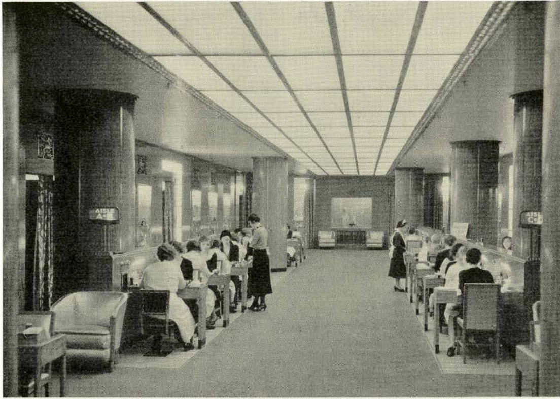
In this hair-dressing salon the entire ceiling becomes the source of light simulating the overcast sky in providing well diffused illumination with a minimum of glare. The lighting is efficient and modern.
