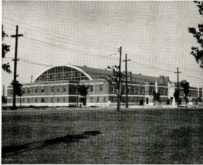
The Fort York Armouries, Toronto . . . another Streamline installation
