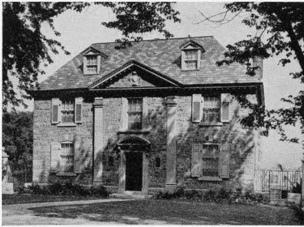
RESIDENCE OF JAS. WILSON, ESQ., WESTMOUNT, P.Q. Perry & Luks, Architects
