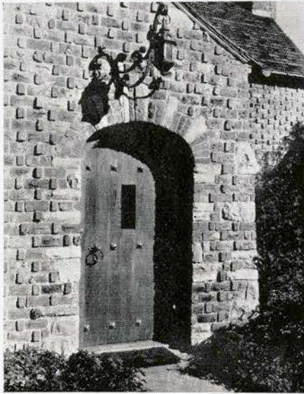
Flemish Bond. The projecting brick headers produce a rough, rugged appearance that places such brick work in the skintled class.
