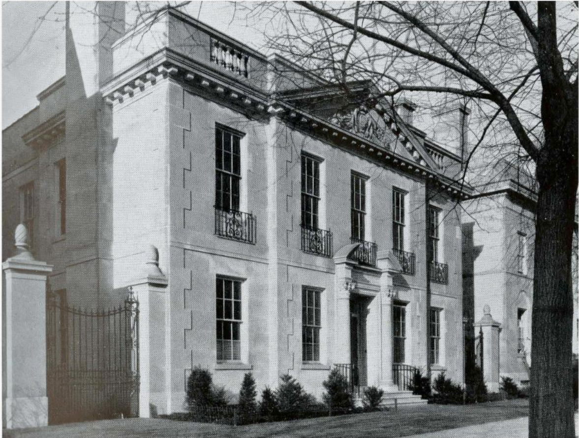
Honourable Mention—Class III—Office Buildings BUILDING FOR PROVINCIAL PAPER LIMITED, TORONTO Marani, Lawson & Morris, Architects
