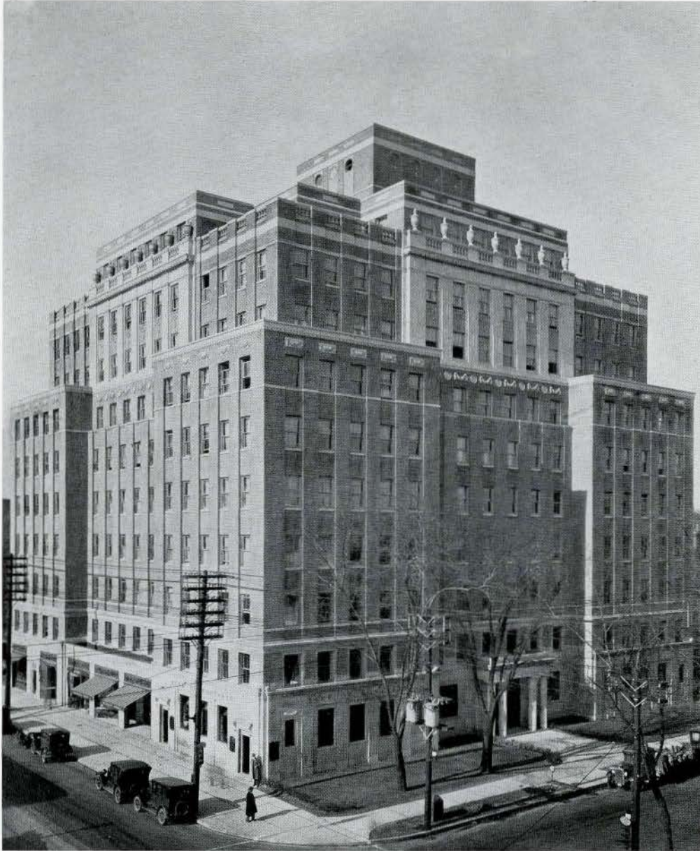
Honourable Mention—Class III—Office Buildings MEDICAL ARTS BUILDING, TORONTO Marani, Lawson & Paisley, Architects
