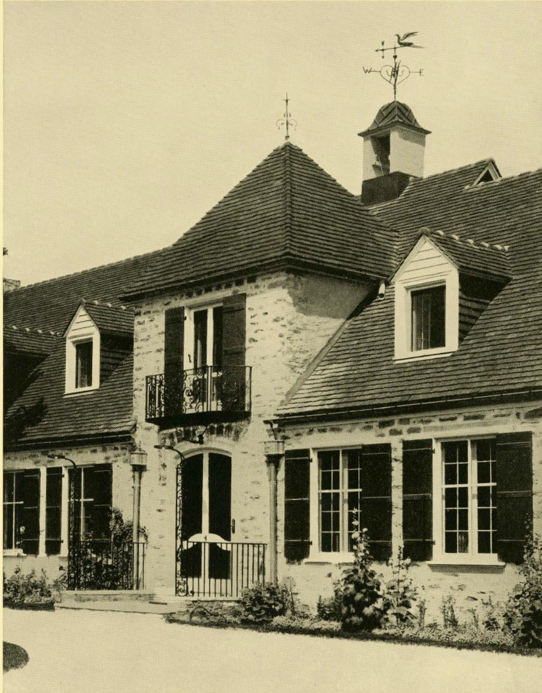
ENTRANCE DETAIL, RESIDENCE OF MRS. A. B. COLVILLE, ST. HENRI DE MASCOUCHE, P.Q.
