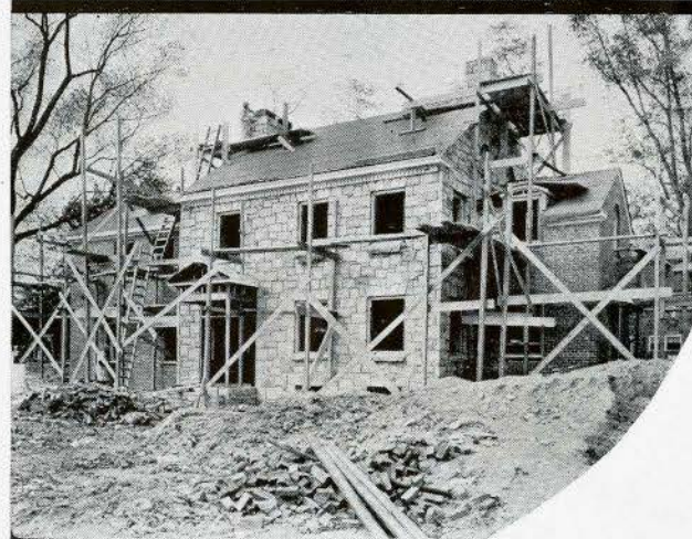
Note brick and stone facing applied over TEN/TEST sheathing.
