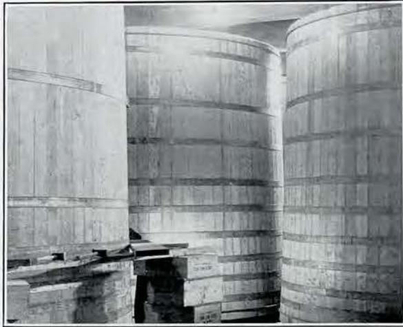
THE ILLUSTRATION SHOWS A BATTERY OF CALIFORNIA REDWOOD TANKS AT A WINERY IN ONTARIO
