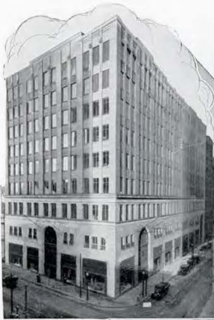
The Robert Simpson Co's. New Building, equipped with Teck Flush Valves. Chapman and Oxley, Architects. Purdy Mansell limited, Plumbing Contractors.
