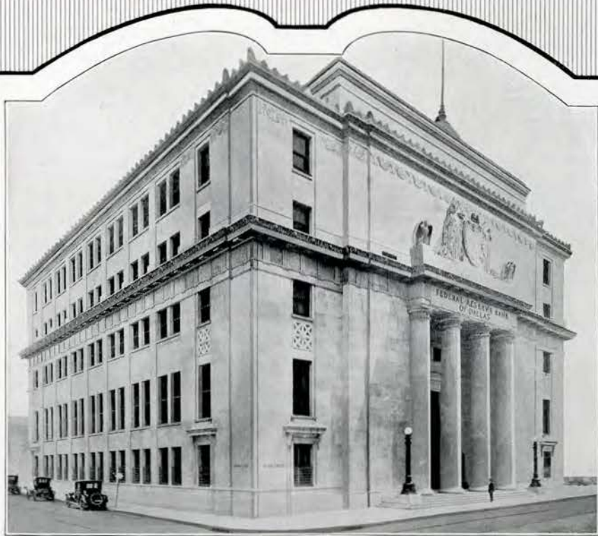
Federal Reserve Bank . . . . . Dallas Graham, Anderson, Probst & White, Chicago, Architects. Mehring & Hansen, Chicago, Heating Contractors
