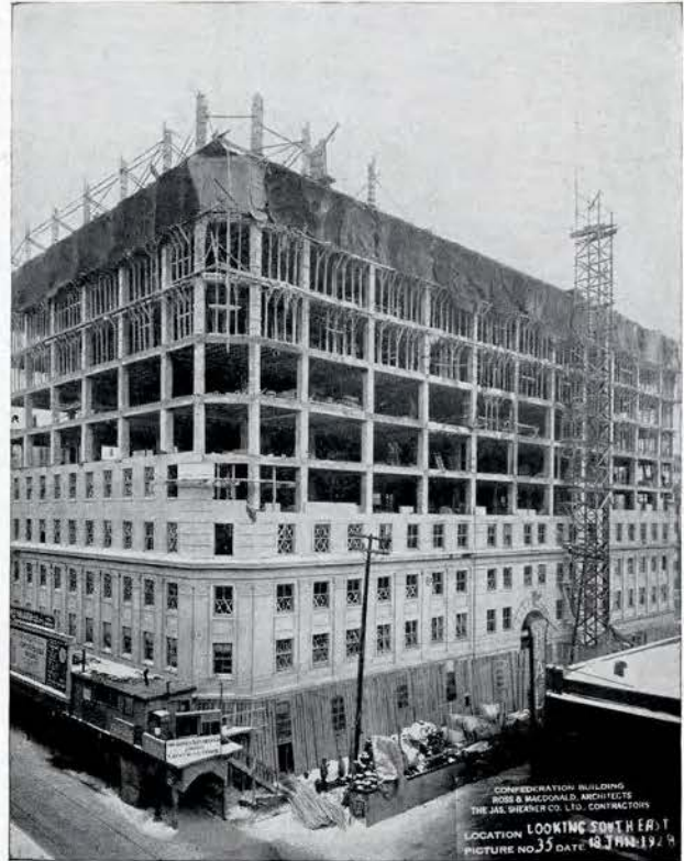
The Confederation Building, Montreal, during construction. Ross & McDonald, Architects; James Shearer Company, Limited, Contractors.
