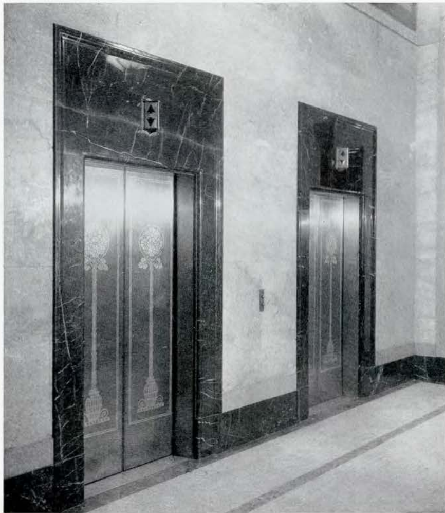
DETAIL OF ENTRANCE TO ELEVATORS
