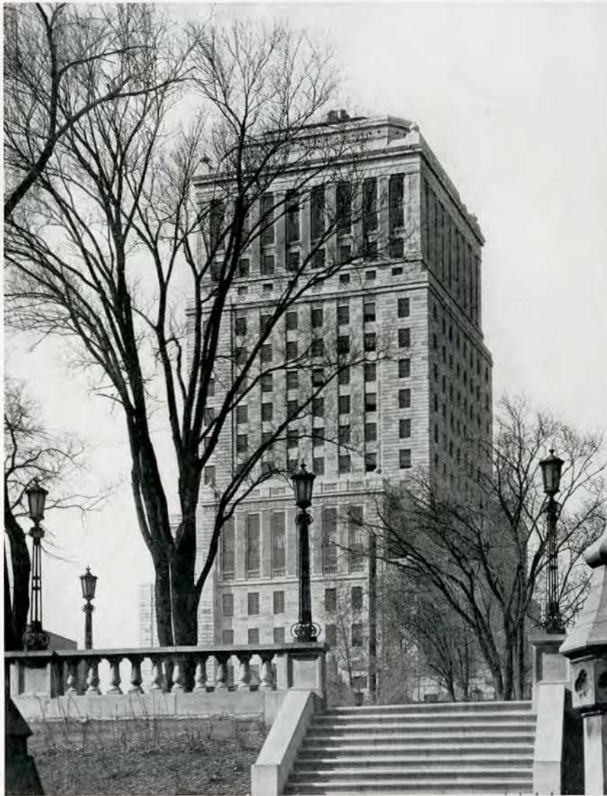
VIEW FROM NORTH-EAST
