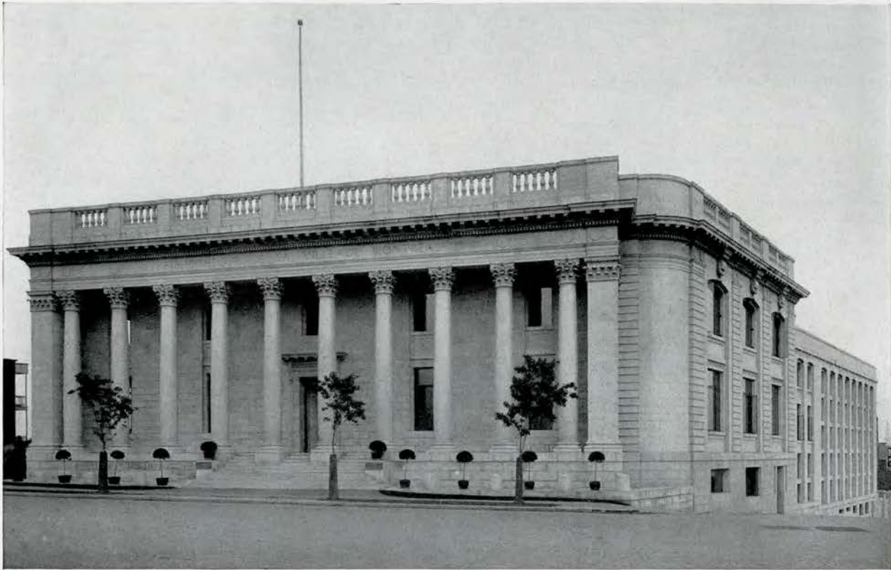
MONTREAL PUBLIC LIBRARY Eugene Payette, Architect
