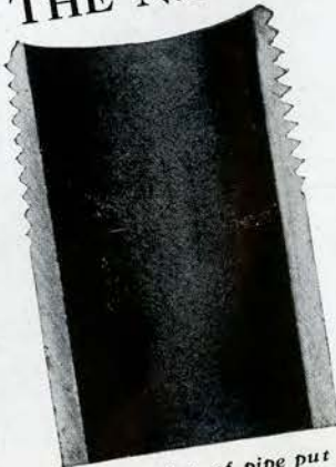
Interior view of pipe cut through the Scale Free Process
