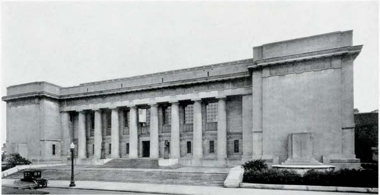
INDIANAPOLIS PUBLIC LIBRARY Paul Cret, Zantzinger, Borie and Medary, Architects
