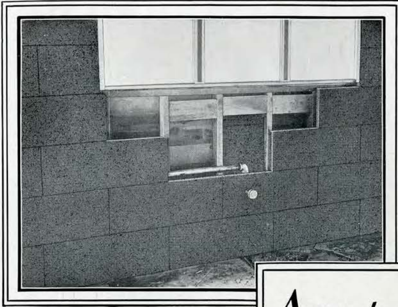
Armstrong's Corkboard applied to the walls of M. J. Schubert's residence, Pierre, S. D.
