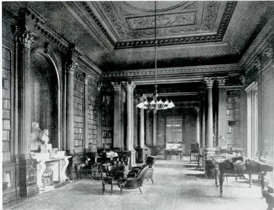
LIBRARY—REFORM CLUB, LONDON, ENGLAND Sir Charles Barry, Architect
