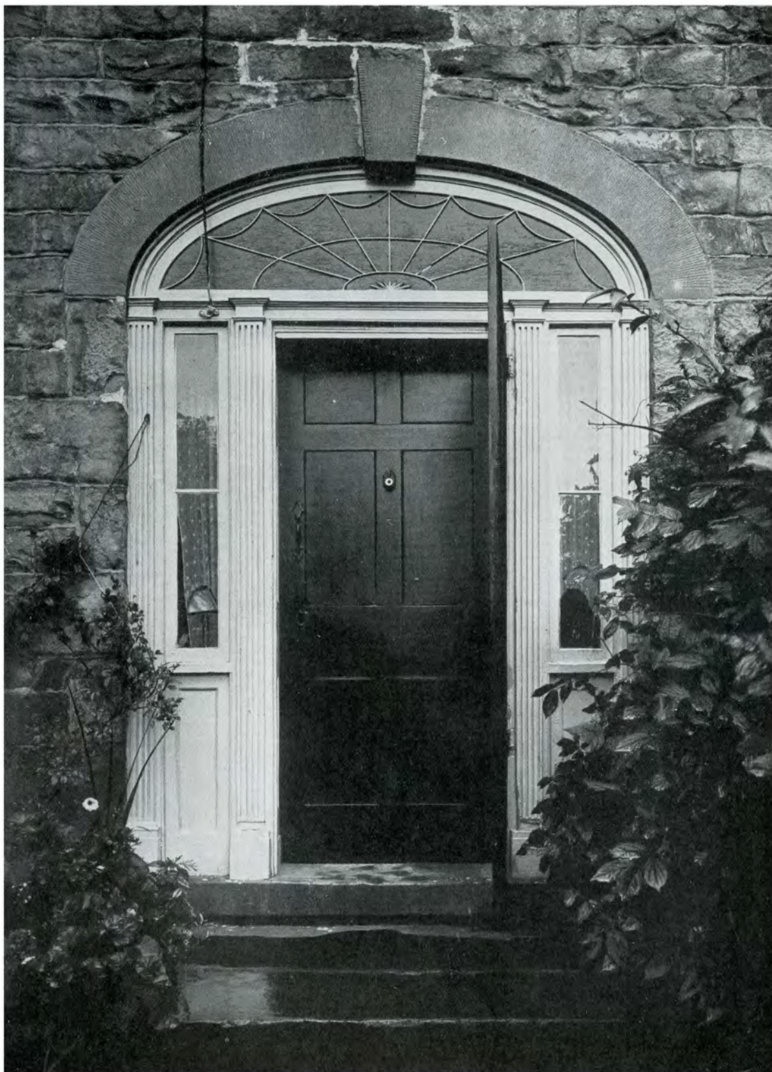
DOORWAY, PREST HOUSE, QUEENSTON, ONT.
