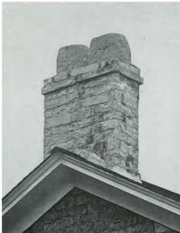
CHIMNEY OF PREST HOUSE, QUEENSTON, ONT.
