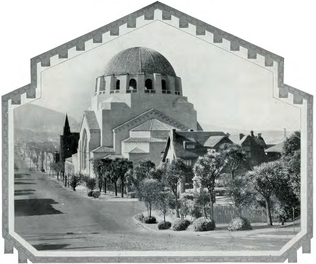
TEMPLE EMANU-EL, SAN FRANCISCO . . . . . EQUIPPED WITH JOHNSON HEAT CONTROL BAKEWELL, BROWN AND SYLVAIN SCHNAITTACHER, . . . . . ASSOCIATED ARCHITECTS
