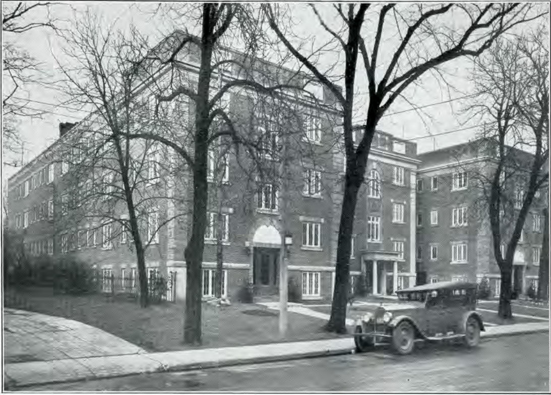
The "Commodore," Toronto, 135 suites—all equipped with Frigidaire. Roberts Construction Co., Toronto
