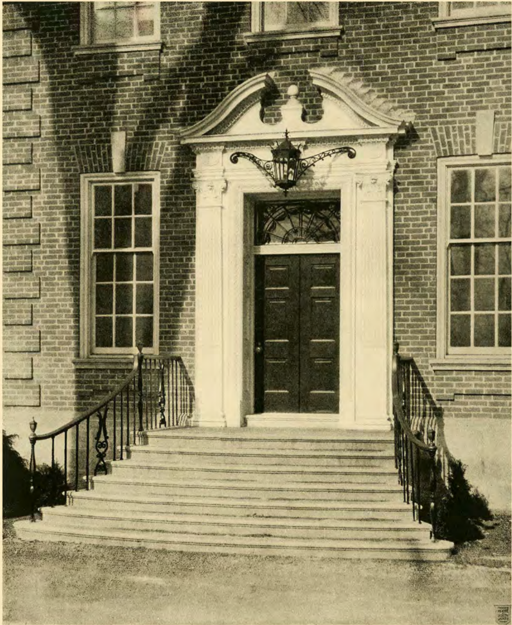
MAIN ENTRANCE DOORWAY, RESIDENCE OF G. R. LARKIN, ESQ., TORONTO George, Moorhouse and King, Architects
