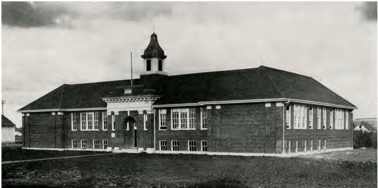
ST. ALPHONSUS R.C. SEPARATE SCHOOL, EDMONTON, ALTA. Edward Underwood, Architect
