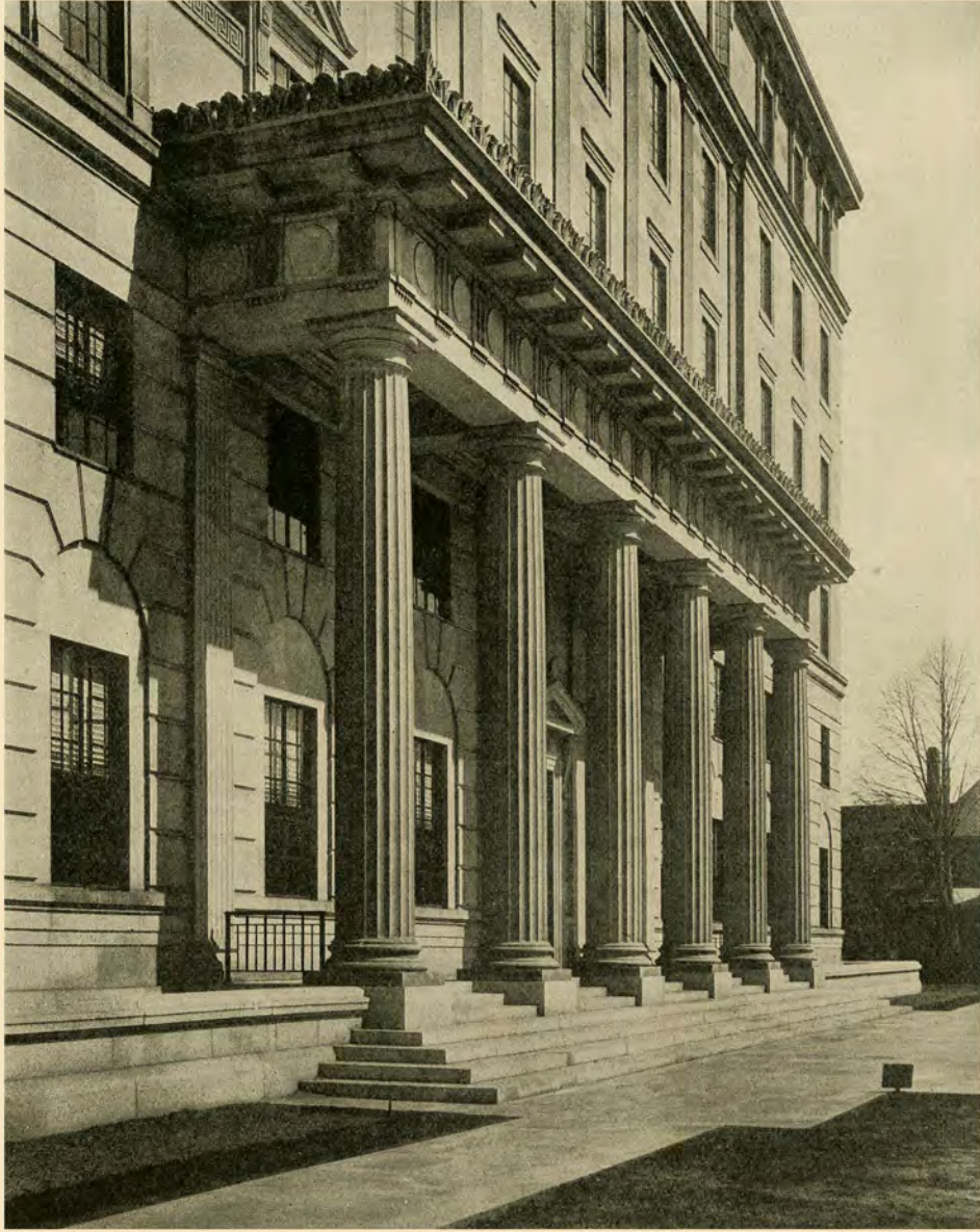
ENTRANCE PORTICO, MANUFACTURERS' LIFE INSURANCE CO., TORONTO Sproatt & Rolph, F.F.R.I.B.A., Architects
