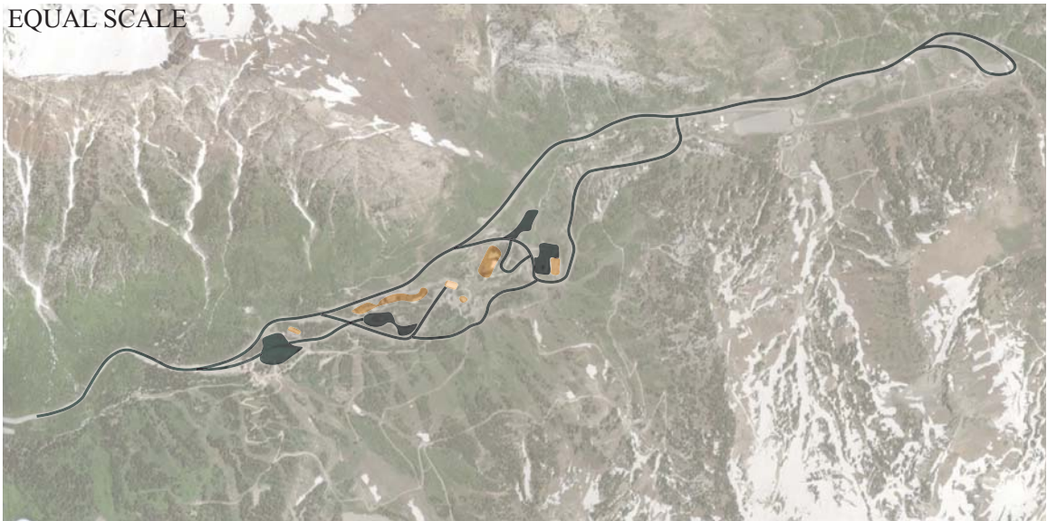
Snowbird Mountain Resort: Architectural developments in yellow and transportation infrastructure in black
