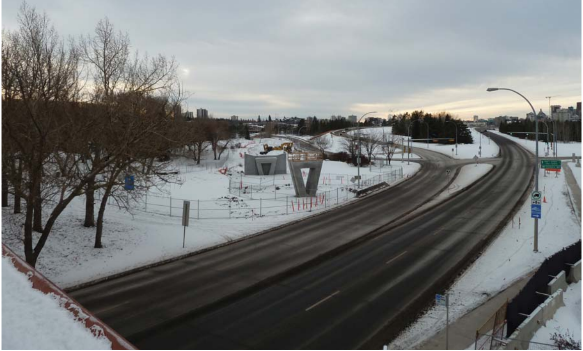
1 - Elevated track infrastructure.
