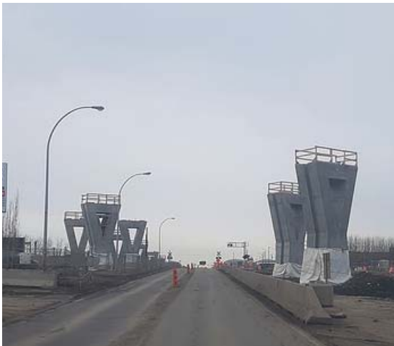
1 - Elevated track infrastructure. Image by Paul Smolik.
