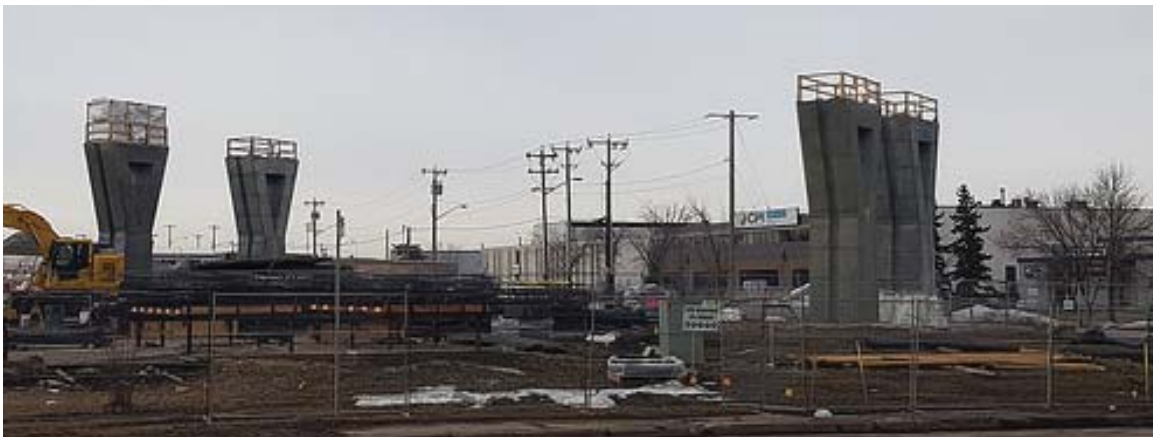
3 - View of station columns. Image by Paul Smolik.
