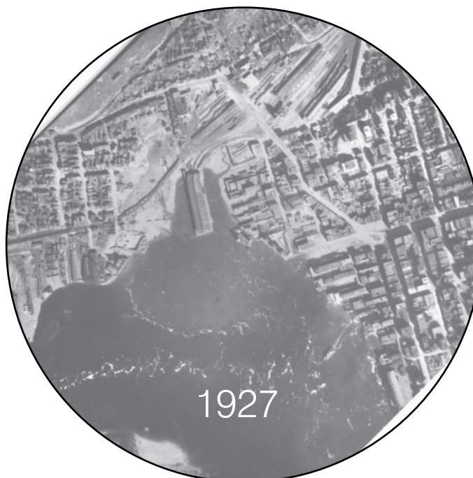
Fig. 7. Aerial Photo of Saint John from 1927. Note the Long Wharf terminal, Portland Point neighbourhood to the west, and dry area caused by the tide being low. Yves Leger [ Manager Geographic Information Systems/ Data Analytics for the City of Saint John] email, September 13 2017.
