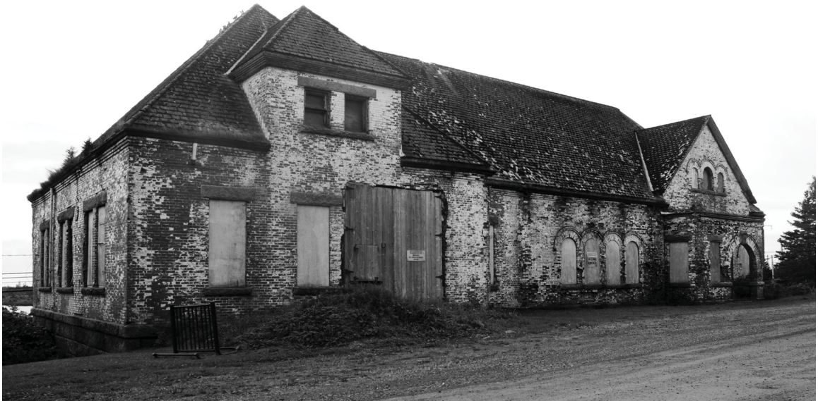
Hazel-Hill Cable Station, photograph, 2016.
