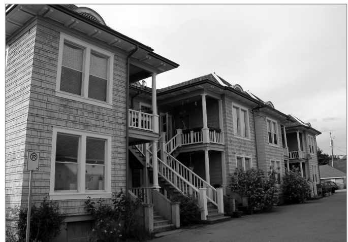
FIG. 24. APARTMENT BUILDING BUILT IN 1916 IN THE TOWN CENTRE OF POWELL RIVER. | LUCIE K. MORISSET.
