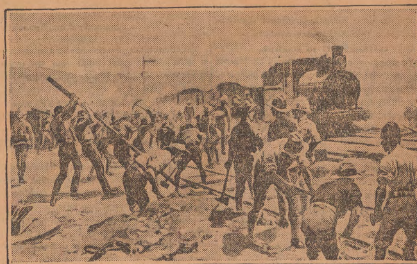
"A knot of sappers came up from the river, where they had been tamping ballast under a new siding."
