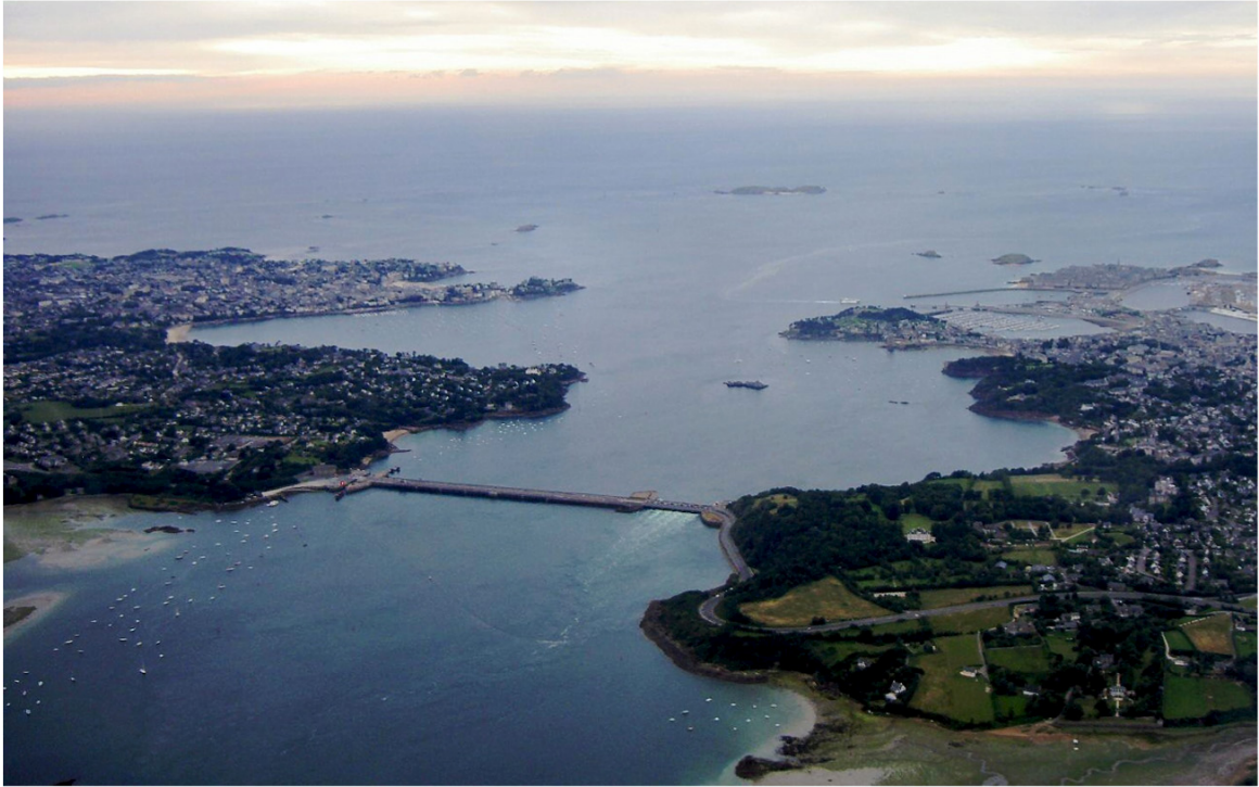
Figure 1-5: Tidal Barrage Power Plant in Rance, France [18]
