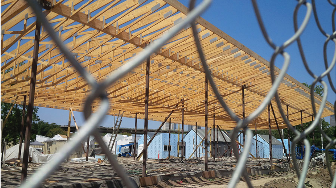
Image of Cottages project under construction
