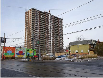
High-rise, low income residential building
