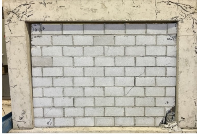
a) Overview of Infilled Frame at Failure
