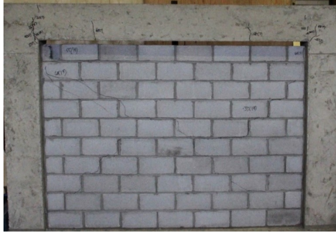
a) Overview of Infilled Frame at Failure
