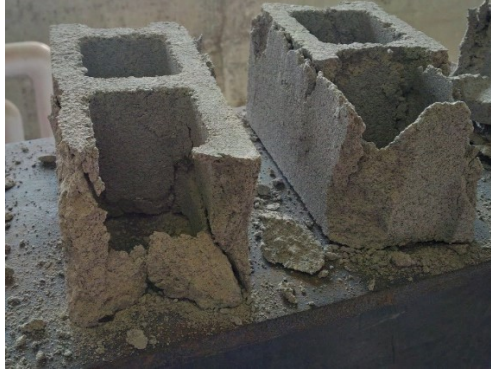
Figure 4.2 Typical Failure Mode of the CMUs
