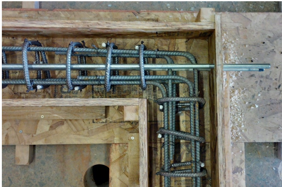
Figure 3.7 Formwork with Reinforcement and Threaded Rod Detail
