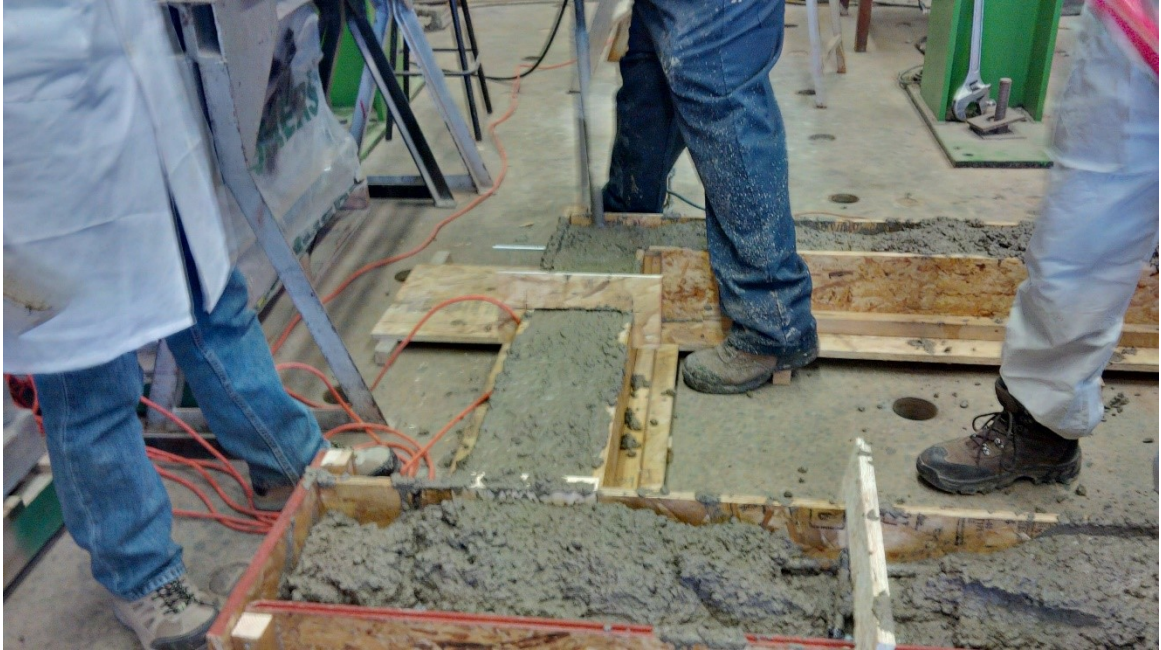
Figure 3.8 Concrete Casting with Vibration
