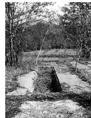
Foundation of truck service station Ribbon Creek; photograph by Johnnie Bachusky
