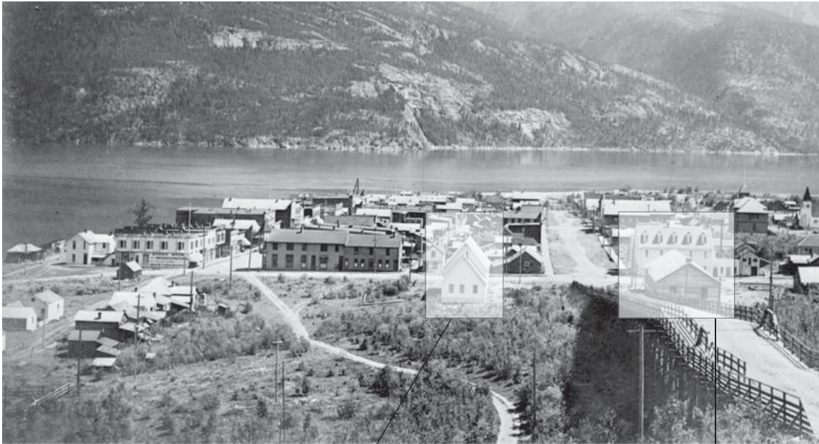
Fig. 46. Trestle and Church Site, 1902; photograph from BC Archives.
