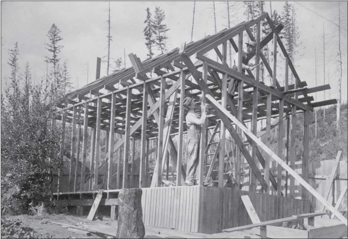
Fig. 12. Wood-Frame Construction in Kaslo, photograph from BC Archives.
