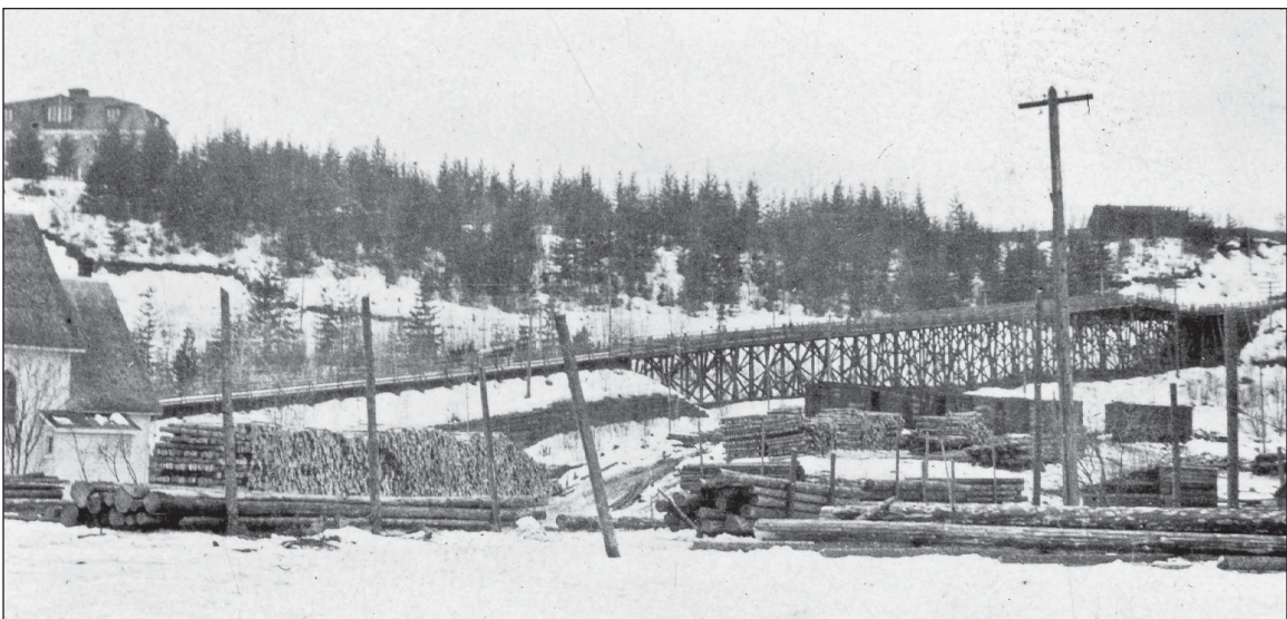
Fig. 49. Trestle Site, early 1900's; photograph from KLHSA.
