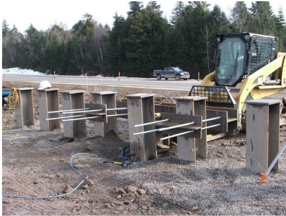
Figure 3.4 Photo of Test Configuration for Static Push Test of Pile P5N.
