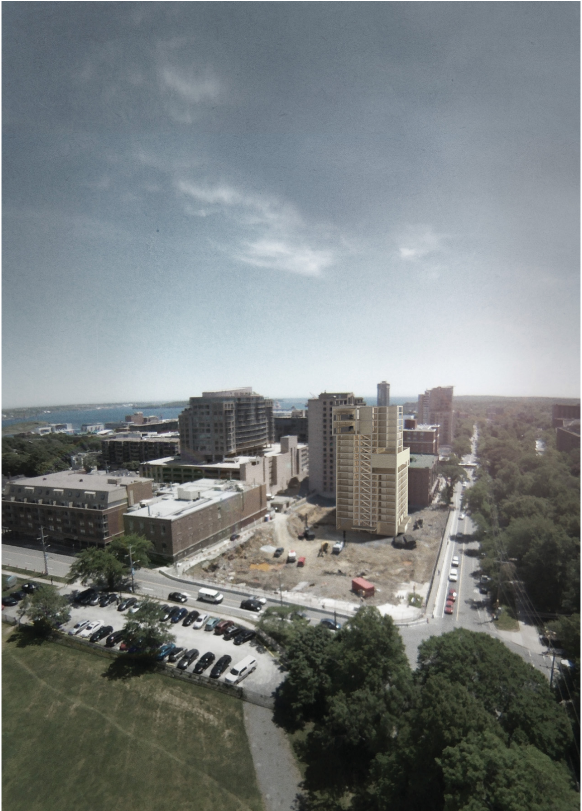
Figure 32. Image showing building structure and site context.
