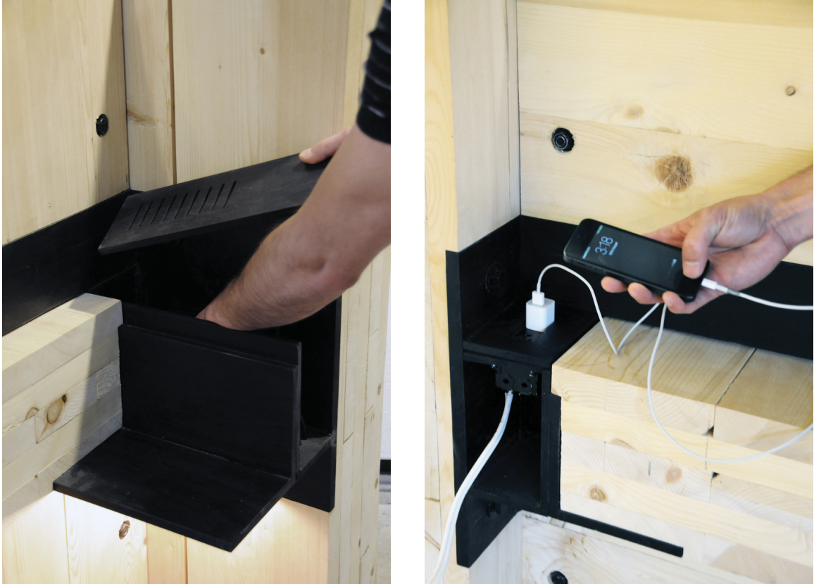
Figure 16a,b. Detail images taken of the 1:1 model showing accessibility and connection to power through the steel system.
