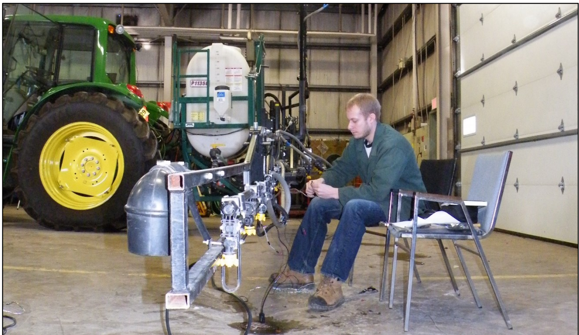
Figure A-5: Wiring individually controlled solenoid valves for each nozzle on smart sprayer.
