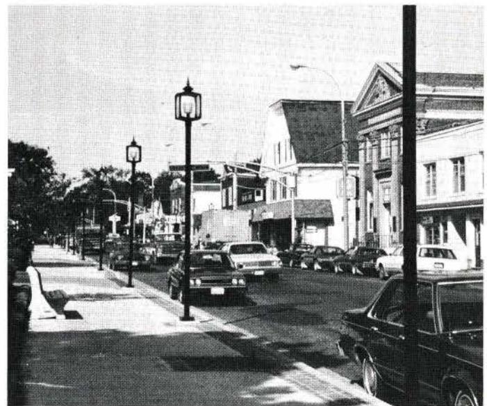
The average town participating in the Program has a population of less than 3,000. Revitalization is phased over a number of years. Here a streetscaping project is nearing completion of year one of a three-year plan.
