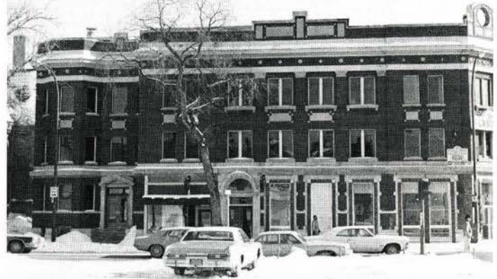
The Courtyard, four levels of boutiques, restaurants and offices, formed the cornerstone for the revitalization of an entire area, now known as Osborne Village.
