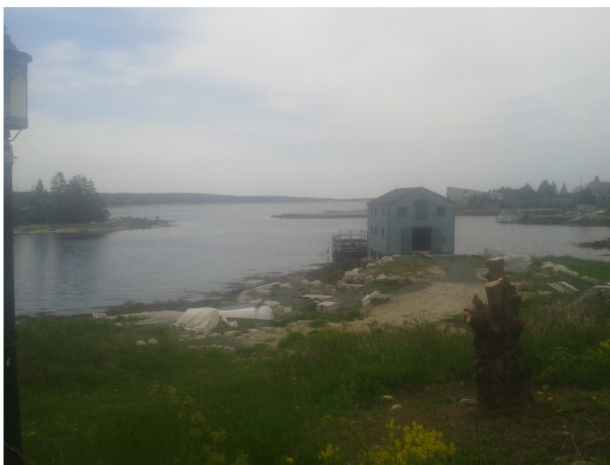
Figure 4.2: Photograph showing protected building at the foot of the cove and stream connecting the Gray Lake-Fawson Cove estuary system pictured to the right of the building. Elevation between the cove and the lake is approximately 5 m.
