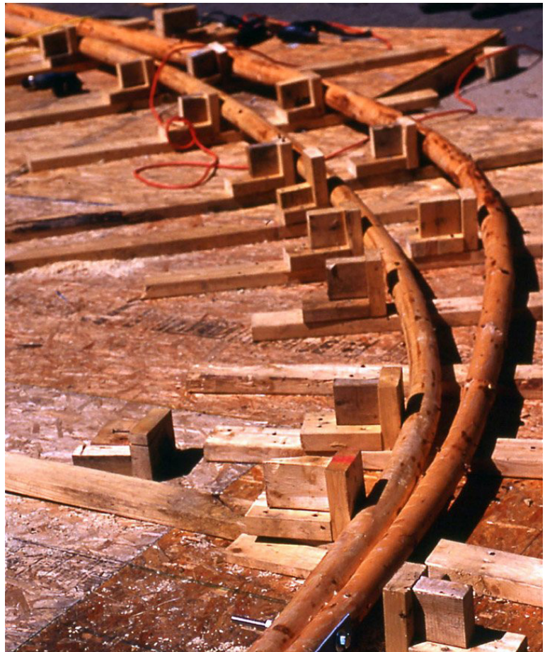
Bentwood truss in assembly using jig blocking system. Image from www.richardkroekerdesign.com
