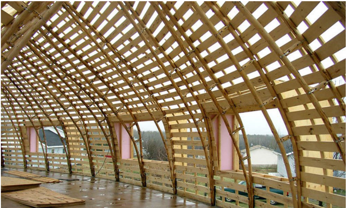
Pictou Landing Health Center under construction, image courtesy of Brian Lilley.
