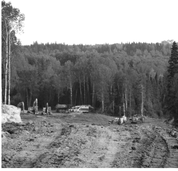
Road construction impacts on the landscape
