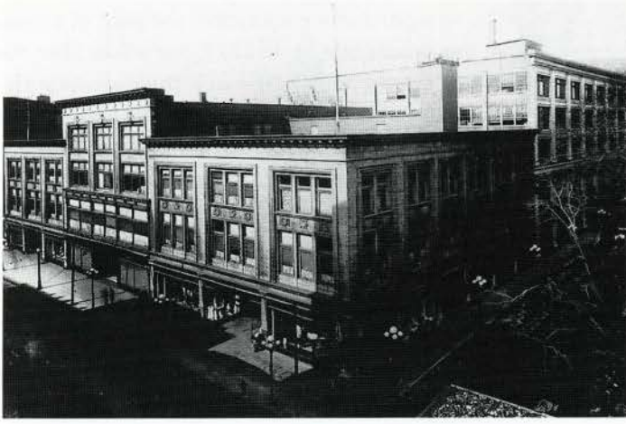
Figure 8. W.H. Scroggie's store, rue Sainte-Catherine, Montreal; architect unknown, 1890; demolished. (Archives of Ontario, Eaton Fonds: AO 4010, F229-308-0-604)
