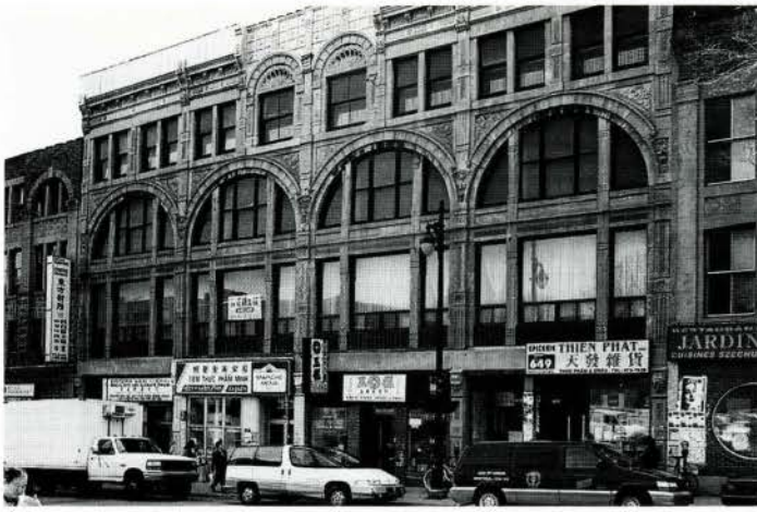
Figure 6. Brunet Building, boulevard Saint-Laurent, Montreal; Daoust & Gendron, architects, 1890. (Gordon Fulton, 1996)
