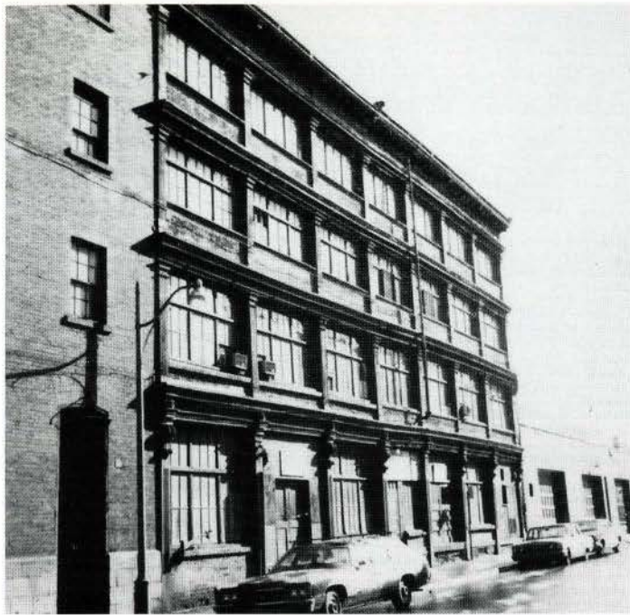
Figure 3. Ives & Allen Company, 261, rue Queen, Montreal; Alexander Cowper Hutchison, architect, 1872. (Canadian Inventory of Historic Building, 1974)
