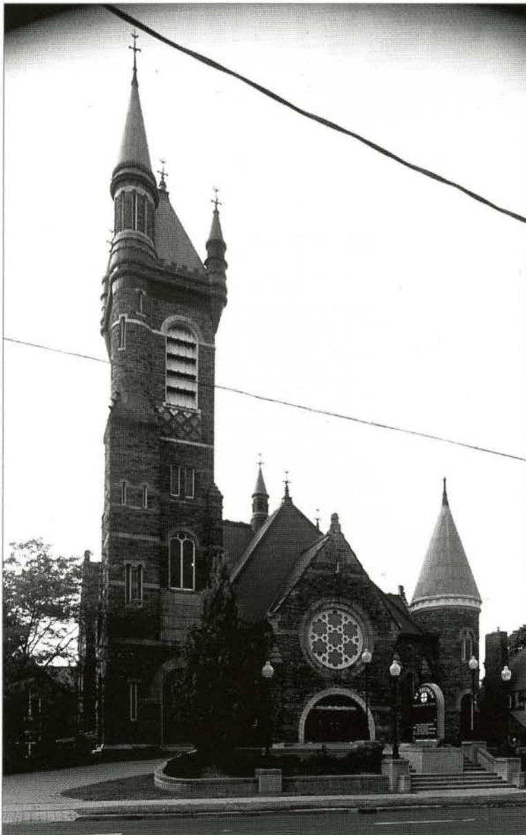
FIG. 1. ST. THOMAS ANGLICAN CHURCH, ST. CATHARINES, ONTARIO, 1877. MILTON EARL BEEBE, ARCHITECT. EXTERIOR, FAÇADE. | Malcolm Thurlby
