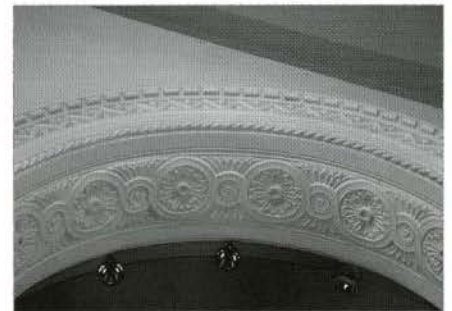
FIG. 15. ST. THOMAS CHURCH, ST. CATHARINES, ONTARIO, 1877. DETAIL OF SOFFIT MOULDING. | Candace Iron.
