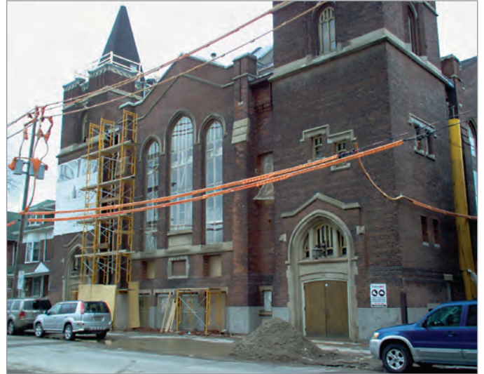
FIG. 7. THE CHURCH LOFTS UNDER CONSTRUCTION. | NICHOLAS LYNCH, 2009.
