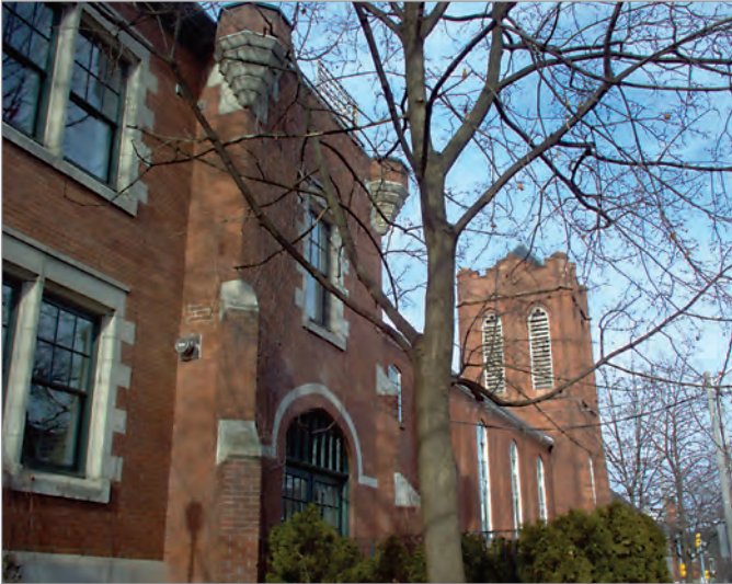
FIG. 6. SOUTHERN ELEVATION OF THE FORMER DOVERCOURT-ST. PAUL'S PRESBYTERIAN CHURCH (C1884), NOW THE "HEPBOURNE HALL LOFTS." | NICHOLAS LYNCH, 2009.
