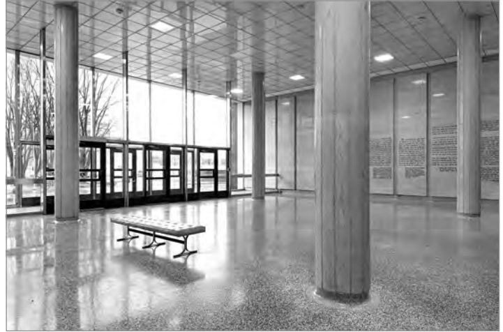
FIG. 9. CENTENNIAL BUILDING MAIN LOBBY, LOOKING TOWARD THE GLAZED STREET ENTRY. NOTE THE TRAVERTINE WALLS AND COLUMNS, TERRAZZO FLOORS, OPAQUE GLASS CEILING, AND PERIOD BENCHES. | MDS PHOTOGRAPHY.
