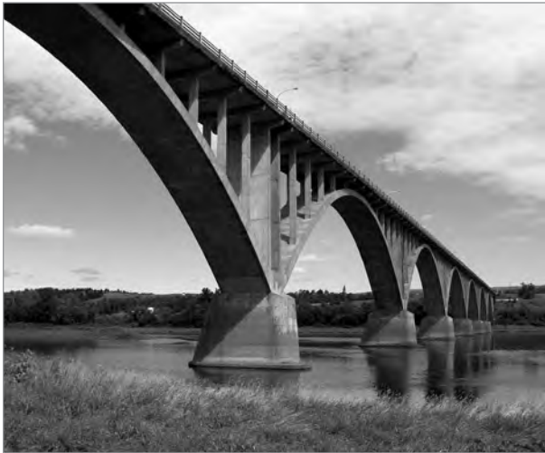
FIG. 2. HUGH JOHN FLEMMING BRIDGE, HARTLAND, NB; COMPLETED 1960. DESIGNER: FOUNDATION OF CANADA ENGINEERING CORPORATION LTD. | JOHN LEROUX.
