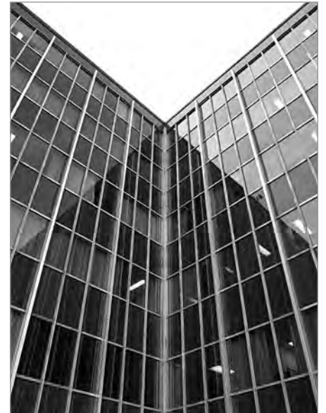
FIG. 7. VIEW OF THE JUNCTION OF THE CENTENNIAL BUILDING'S MAIN WINGS, SHOWING THE PLATE GLASS AND BLACK SPANDREL CURTAIN WALL FACADES, STAINLESS STEEL MULLION FRAMING GRID, AND THE REFLECTIVE QUALITIES OF THE EXTERIOR. | JOHN LEROUX.
