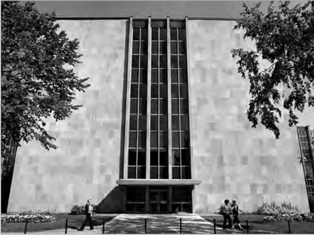
FIG. 8. VIEW OF THE CENTENNIAL BUILDING'S REAR FACADE, WITH ITS PATTERNED SANDSTONE BLOCK CLADDING SURROUNDING A TRIPARTITE VERTICAL SET OF CURTAINWALL GLAZING AT THE HALLWAY ENDS, ABOVE A CANOPIED ENTRY. | JOHN LEROUX.
