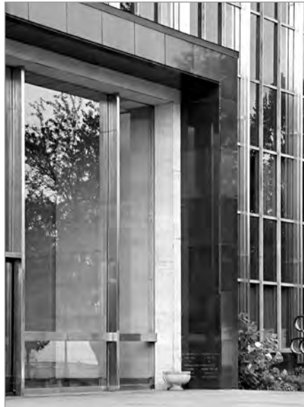
FIG. 6. THE CENTENNIAL BUILDING'S TWO-STOUREY MAIN ENTRANCE INCLUDES A RICH VARIETY OF MATERIALS, INCLUDING POLISHED NEW BRUNSWICK BLACK GRANITE, STAINLESS STEEL WINDOW FRAMING, A REFLECTIVE GLASS CURTAIN WALL, AND TRAVERTINE MARBLE LINING THE LOBBY WALLS. | JOHN LEROUX.
