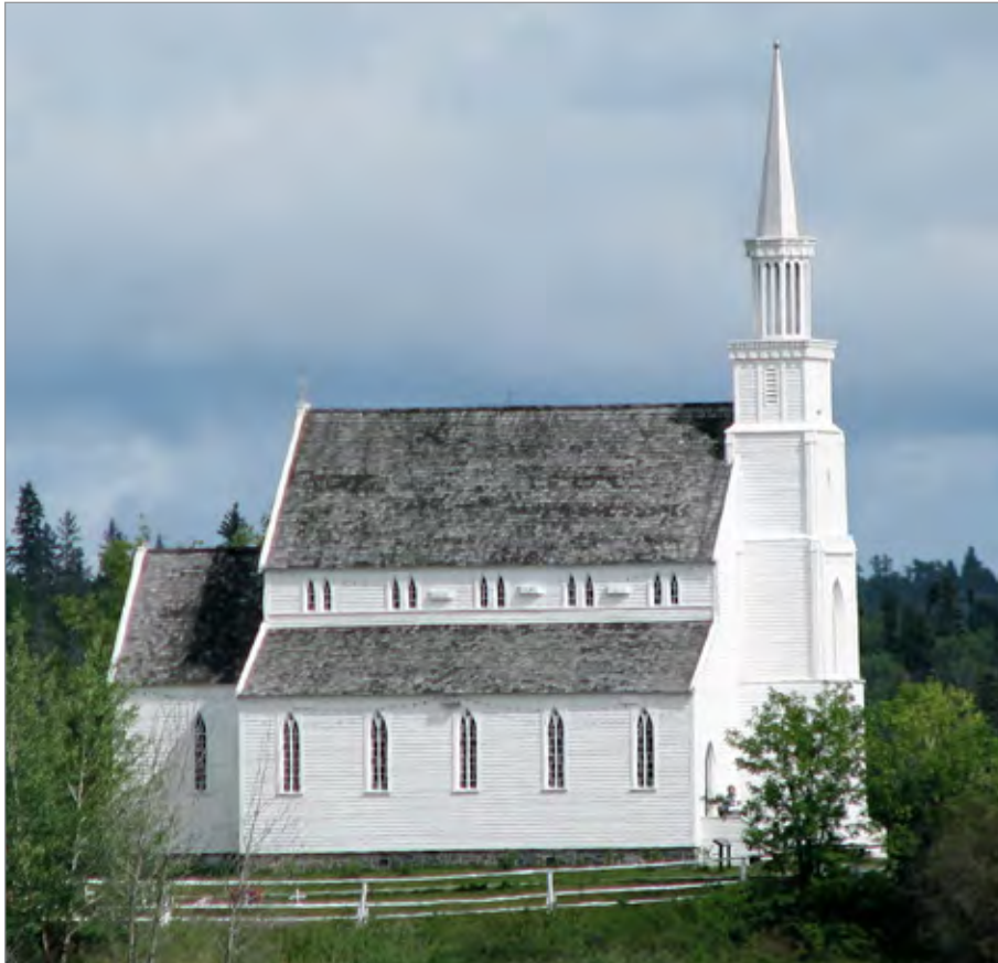
FIG. 2. SOUTHERN SIDE OF HOLY TRINITY ANGLICAN CHURCH, STANLEY MISSION (SK), 1854-1860, ARCHITECT UNKNOWN. | KRISTIE DUBÉ.
