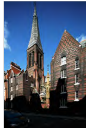
FIG. 10. ALL SAINTS MARGARET STREET ANGLICAN CHURCH, LONDON, ENGLAND, 1849-1859, ARCHITECT WILLIAM BUTTERFIELD. | MALCOLM THURLBY.
