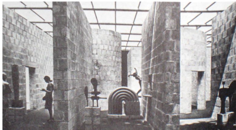
Sonsbeek Pavillion, Sonsbeek Park, Arnhem, Netherlands, 1966. The temporary pavillion was composed of 6 walls 4m high with semi circular punctuations creating spaces for the sculpture gallery, 2013; Socks-Studio.
