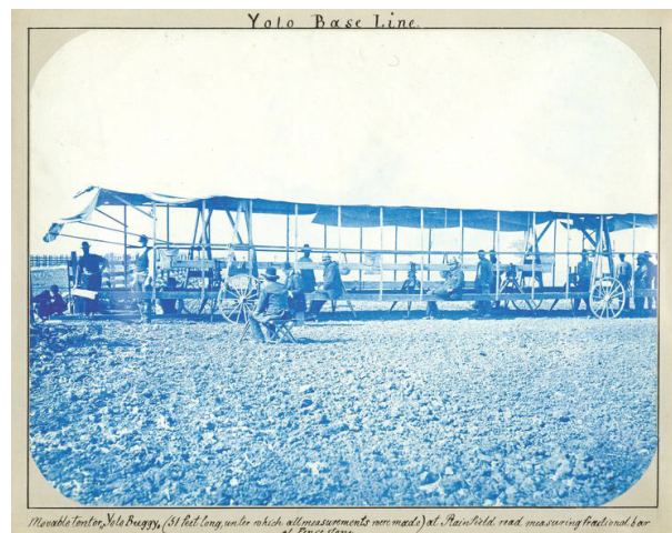
Two historical photographs of the mobile survey apparatus, the “Yolo Buggy”, 2014; Bldg Blog.
