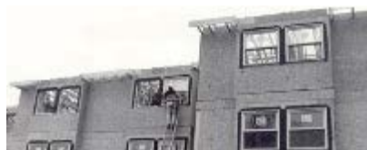
New 80-Bed Women's Residence Under Construction, May 6, 1987
