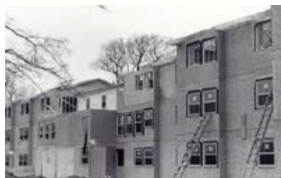
New Women's Residence Under Construction, May 6, 1987
