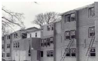
New Women's Residence Under Construction, May 6, 1987
