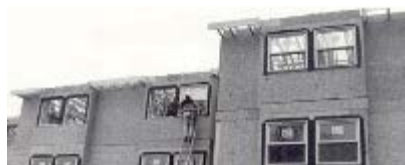
New 80-Bed Women's Residence Under Construction, May 6, 1987
