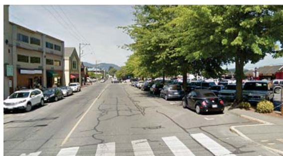
Wide roadways and excessive parking in the downtown area of Duncan. Google Maps
