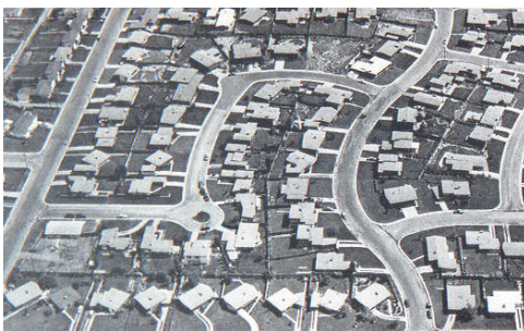
Fig. 12 Aerial view of Arapahoe Acres representing a new pattern of residential development. All houses were oriented on an angle to the street to allow direct views of the Rocky Mountains and to ensure neighbouring houses do not look directly into each other. (Denver Public Library Digital Collections)
