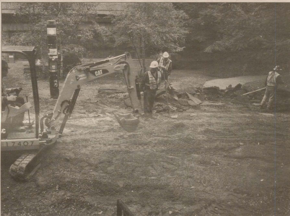
Men working behind the Killam Library on Oct. 10
