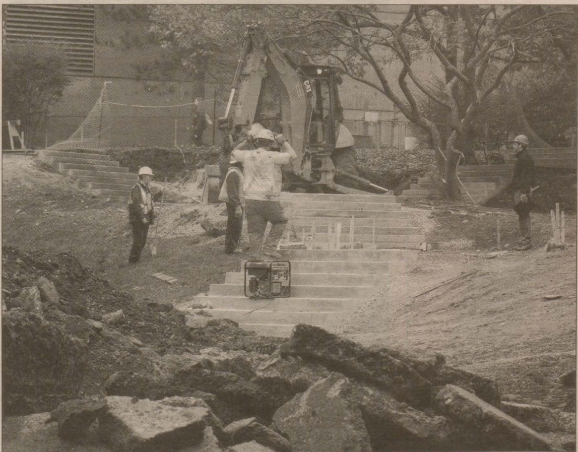
Men working next to the Killam on Oct. 10.
