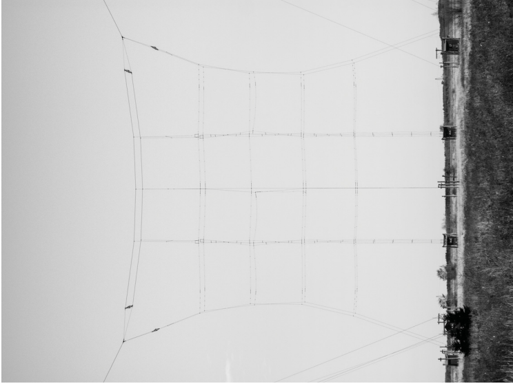
Photos taken mere months before the station's demolition emphasize the sharp contrast of the tall towers in relationship to the expansive landscape. Towers, secured by a sea of guy wires, suspend massive bidirectional antennas. Spacers between each antenna create a tall and slender three dimensional space. Small huts containing the antennas polarity switch boxes scatter the landscape and act as scaling devices for the vast network above.
