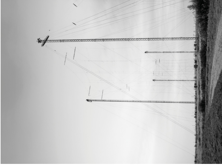
Photos taken mere months before the station's demolition emphasize the sharp contrast of the tall towers in relationship to the expansive landscape. Towers, secured by a sea of guy wires, suspend massive bidirectional antennas. Spacers between each antenna create a tall and slender three dimensional space. Small huts containing the antennas polarity switch boxes scatter the landscape and act as scaling devices for the vast network above.
