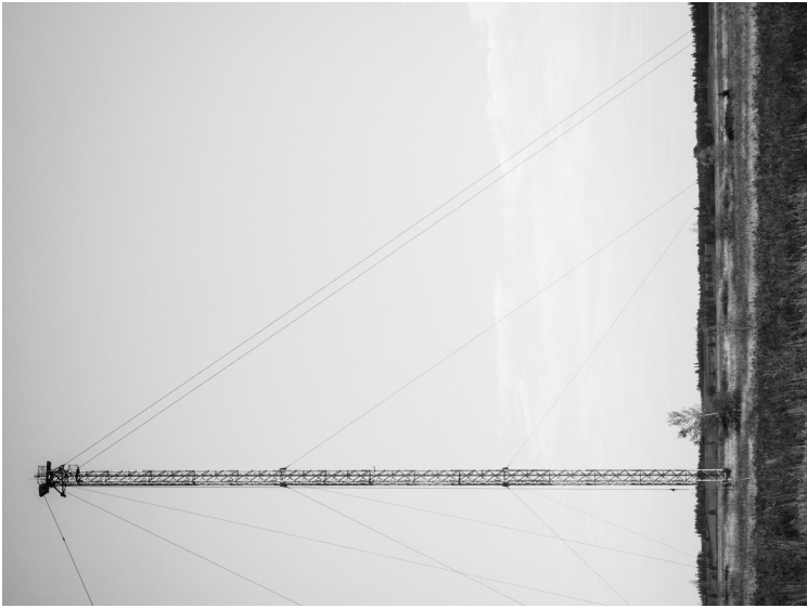
Photos taken mere months before the station's demolition emphasize the sharp contrast of the tall towers in relationship to the expansive landscape. Towers, secured by a sea of guy wires, suspend massive bidirectional antennas. Spacers between each antenna create a tall and slender three dimensional space. Small huts containing the antennas polarity switch boxes scatter the landscape and act as scaling devices for the vast network above.
