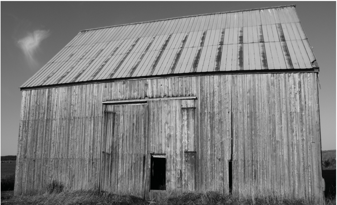
Hay storage barns scattered throughout the Tantramar Marsh act as scaling devices in the landscape. Vertical boards clad these simple structures, providing both light and ventilation.
