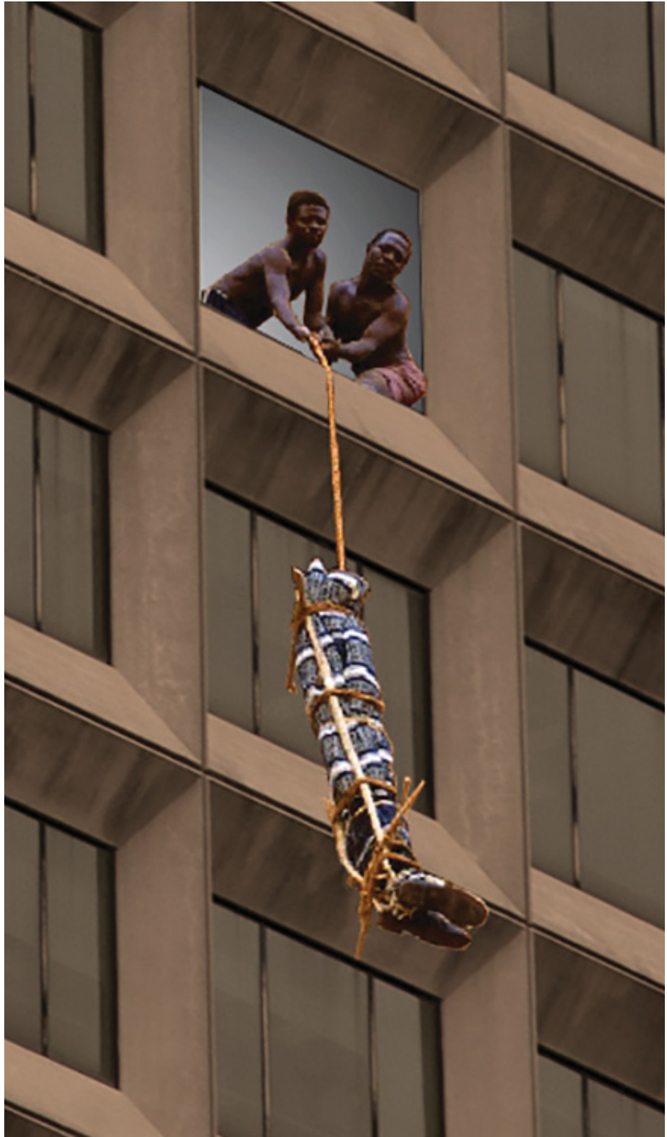
The Bell Aliant office tower has a niche like facade, reminiscent of the caves in the Bandiagara cliffs of Mali where the Dogon bury their dead.
